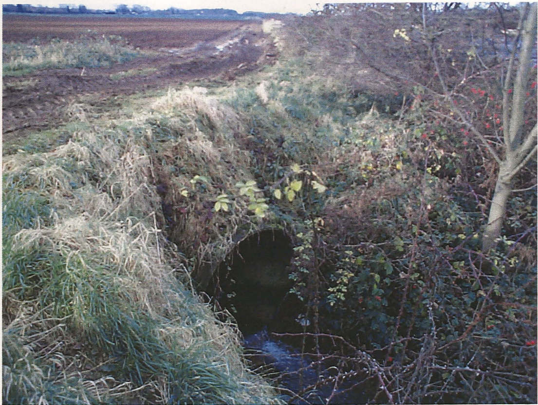
Plate 5 Pipeline Crossing Field Drain
