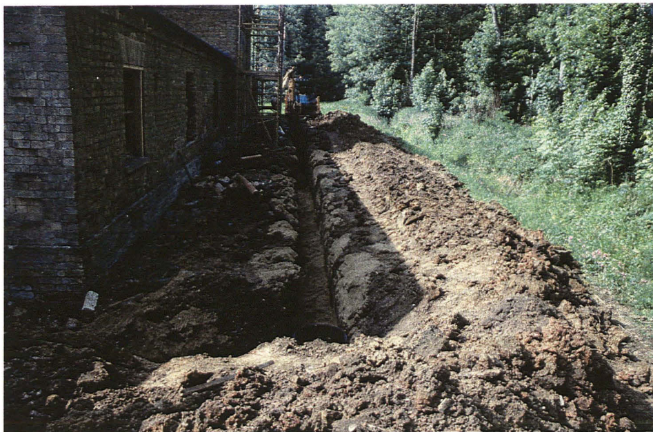
Plate 3 View along main drainage channel, looking north
