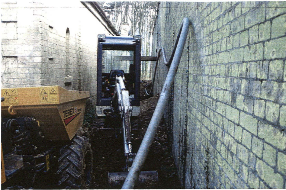
Plate 1 View of drain run under excavation, looking northeast
