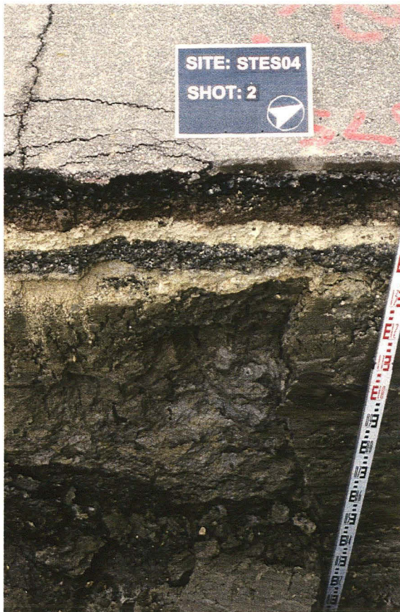
Plate 2 - Section 1, looking west
