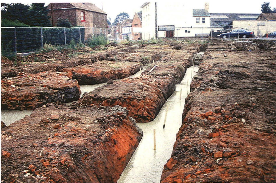
Plate 9 General view of concreted footings, looking West
