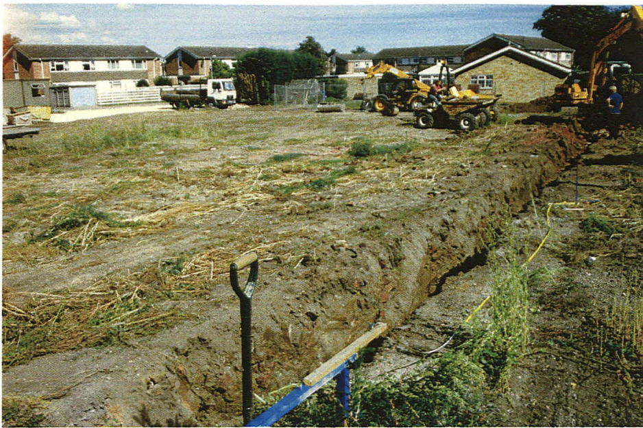
Plate 1 General view of first footings, looking East
