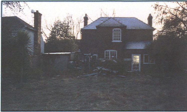
Plate 1 (left): General shot of the development area during machining, looking SE towards the rear of the current house.
