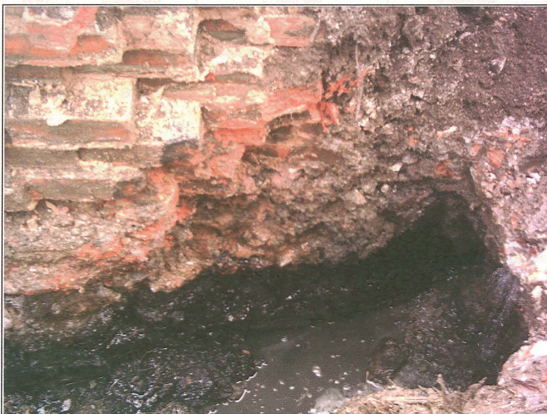
Plate 1: Trial Pit 48 (looking south). Note the grey/black organic layer ([148]) lying at the base of the retaining walls brick foundations.
