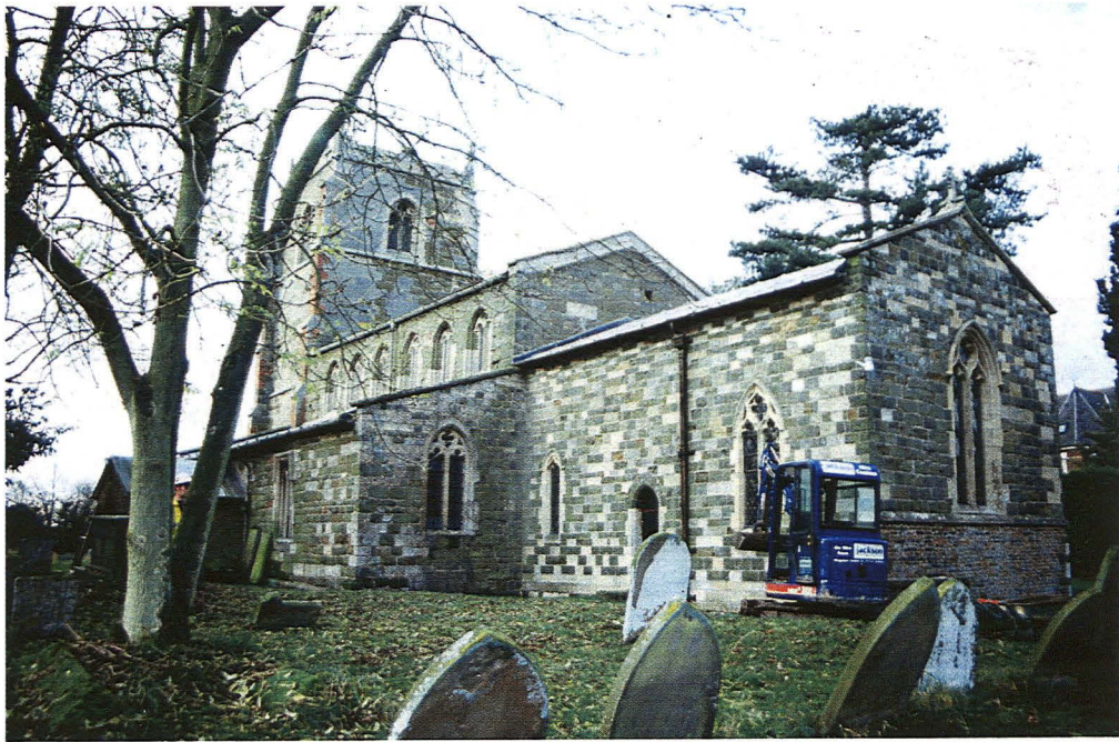
Plate 1 General view of All Saints Church and excavator
