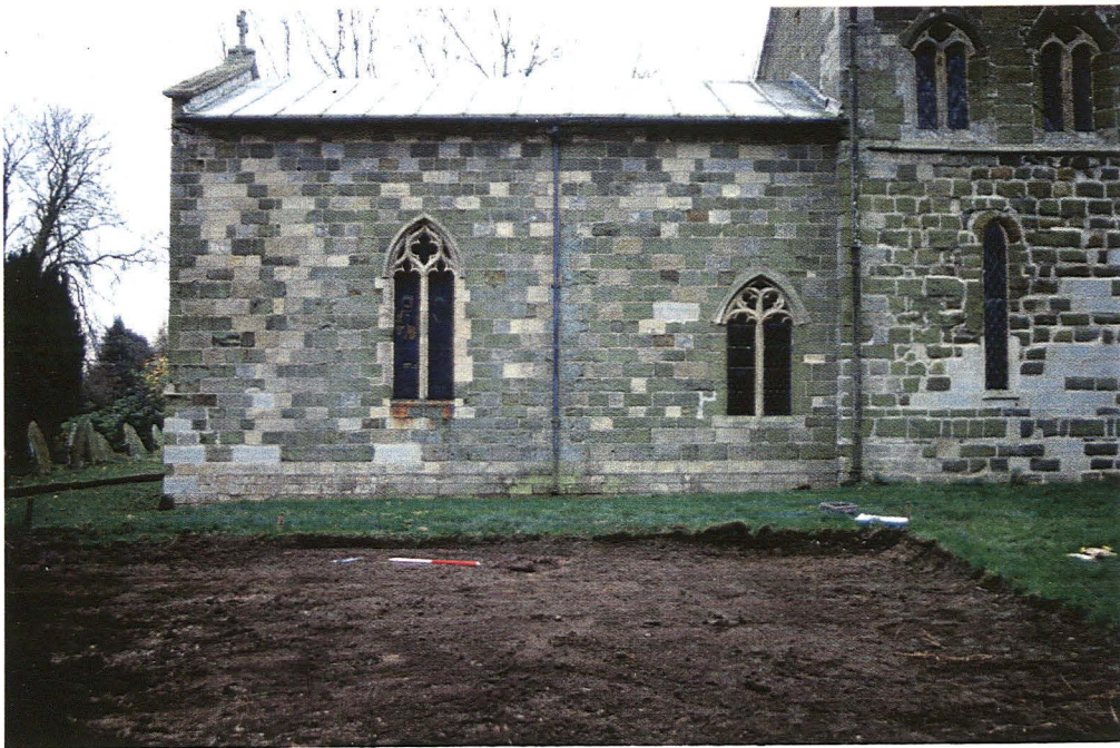
Plate 4 View of East side of church and stripped car park area
