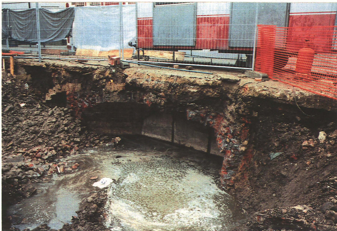
Photo. 9 View of cellar blocking [10] after demolition, looking west
