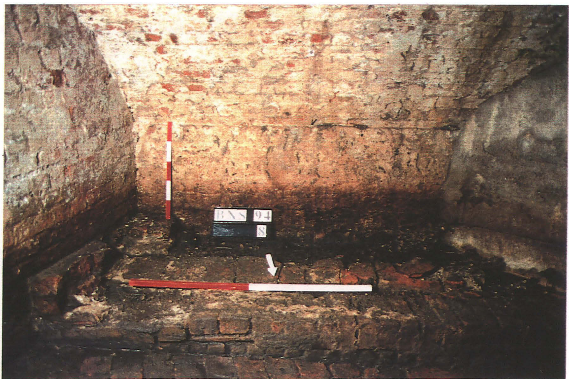
Photo. 4 Looking south at wall elevation [8], with raised brick/tile feature [9] in foreground
