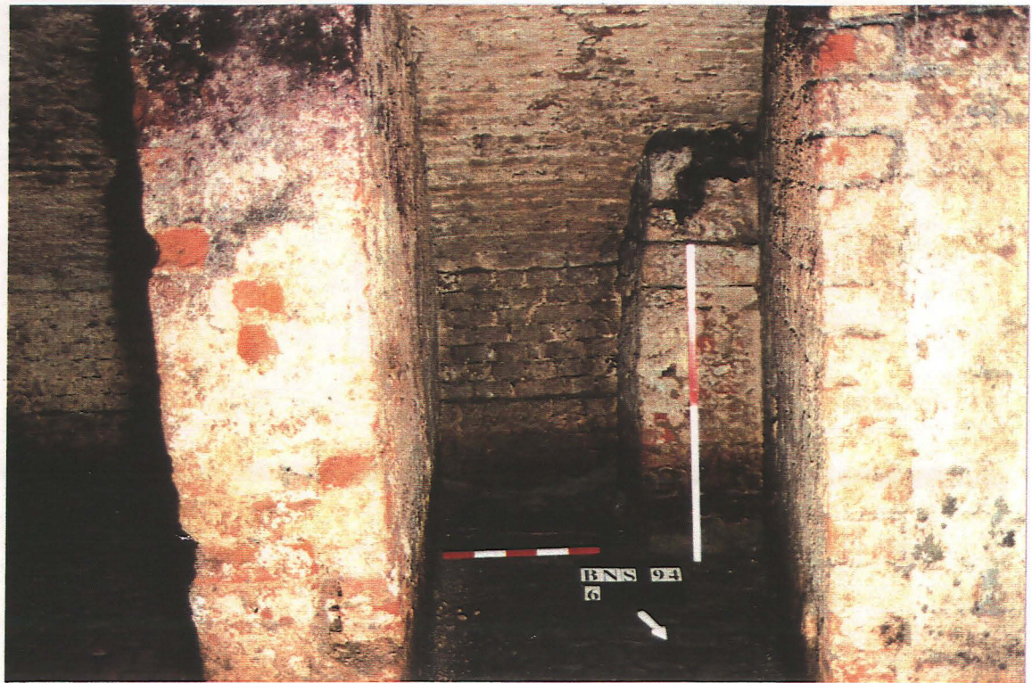
Photo. 3 Looking south-west into small bay demarcated by cross-walls [5] and [7]. Buttress-type feature [6] in right hand corner
