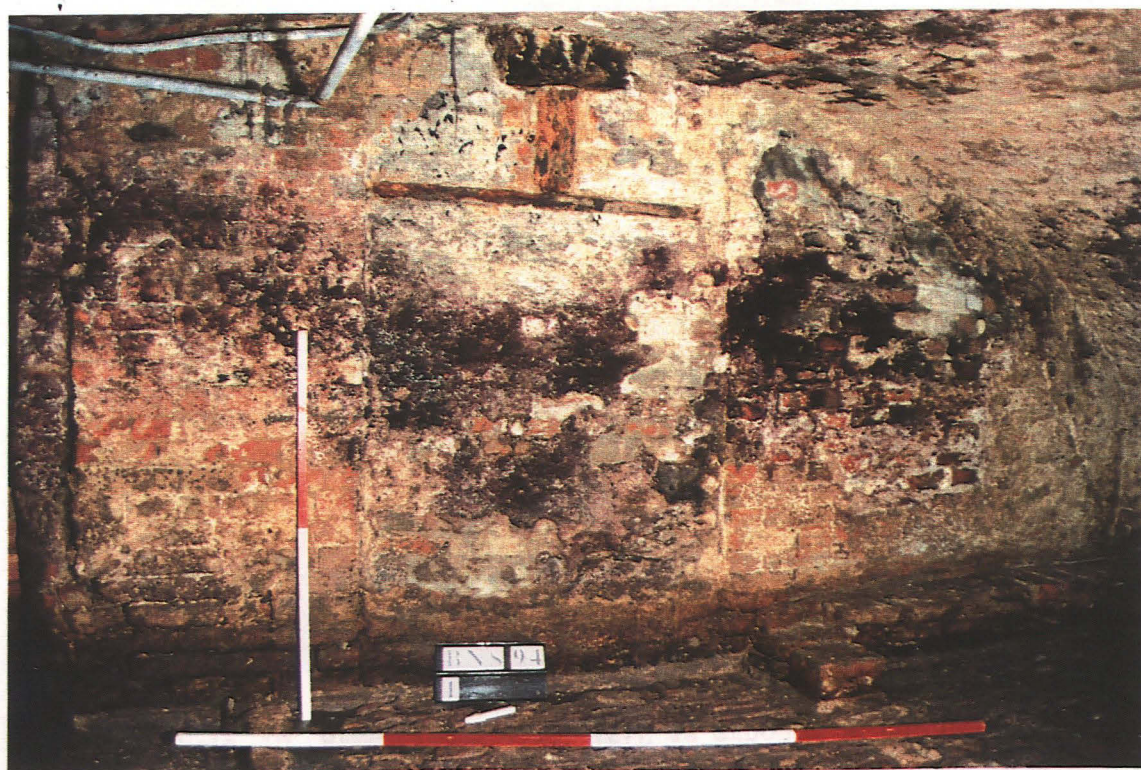
Photo. 8 Looking south-east at south-east elevation of vaulted cellar; incorporating wall [1] and original (blocked) doorway [2]
