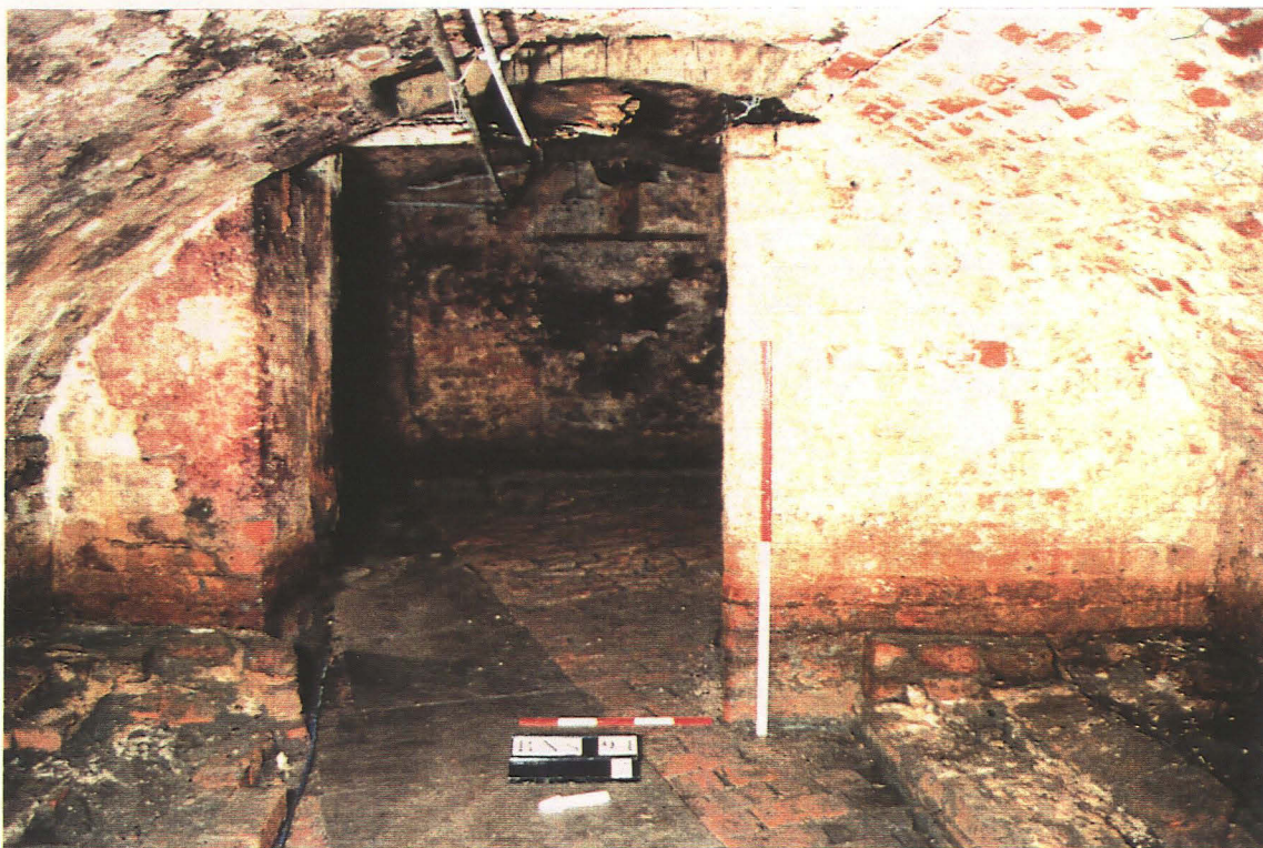
Photo. 1 Looking east from west bay, with cross-wall [7] in foreground
