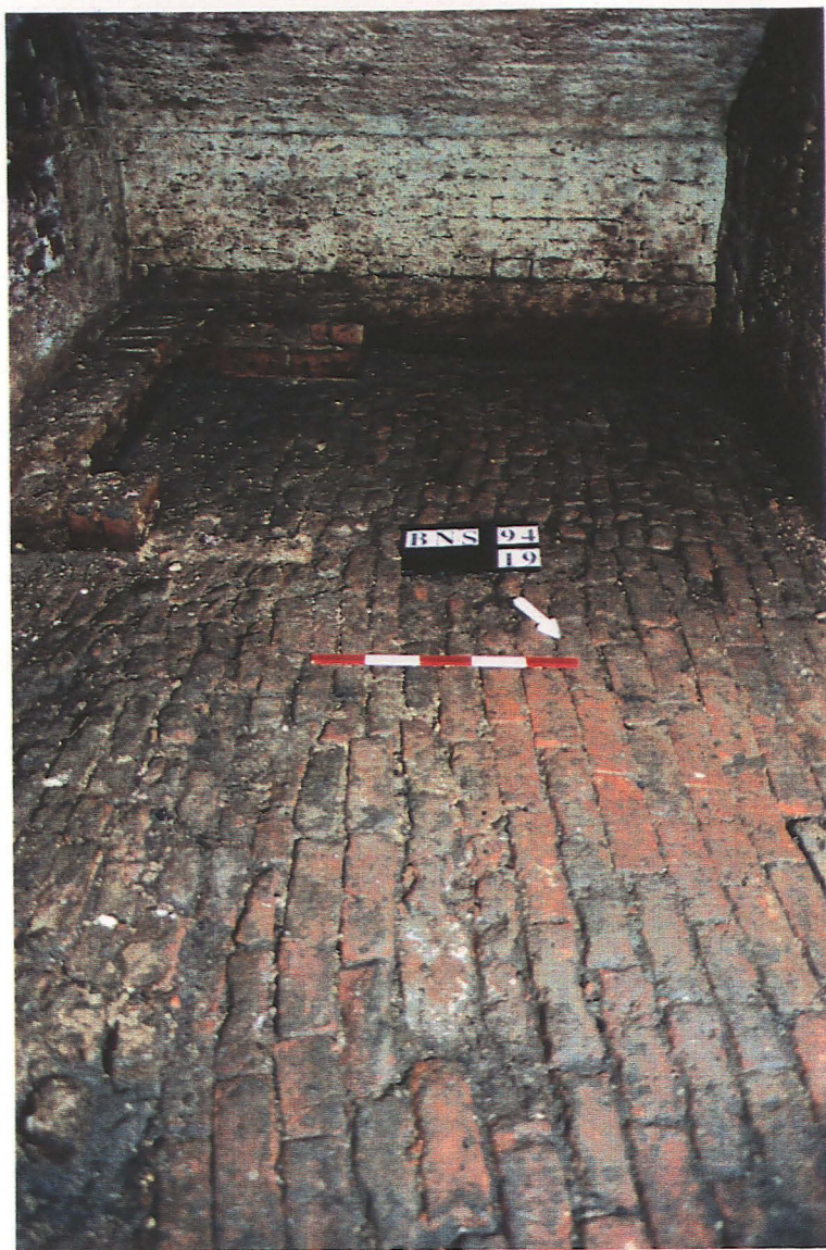
Photo. 7 Looking south-west at brick floor [19] (foreground) and wall elevation [4] (background)
