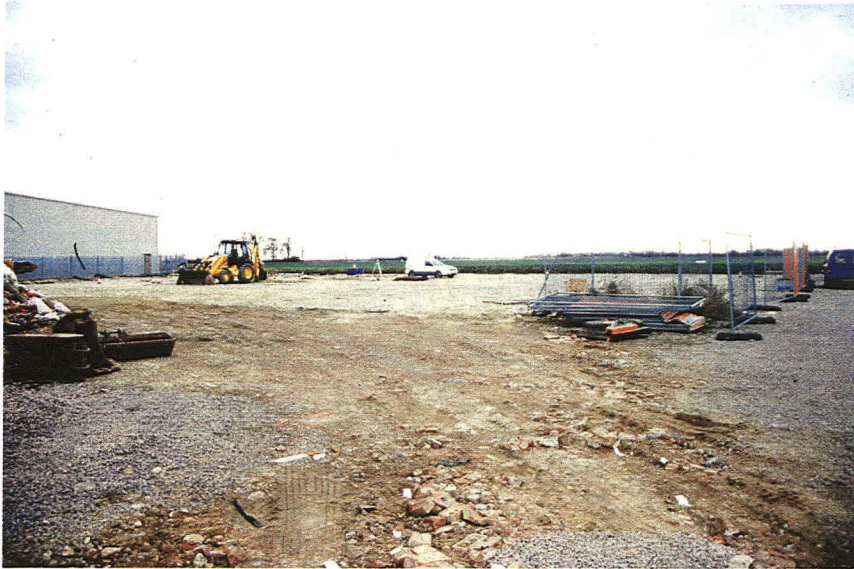
Plate 1 - General view across the development area, looking northwest
