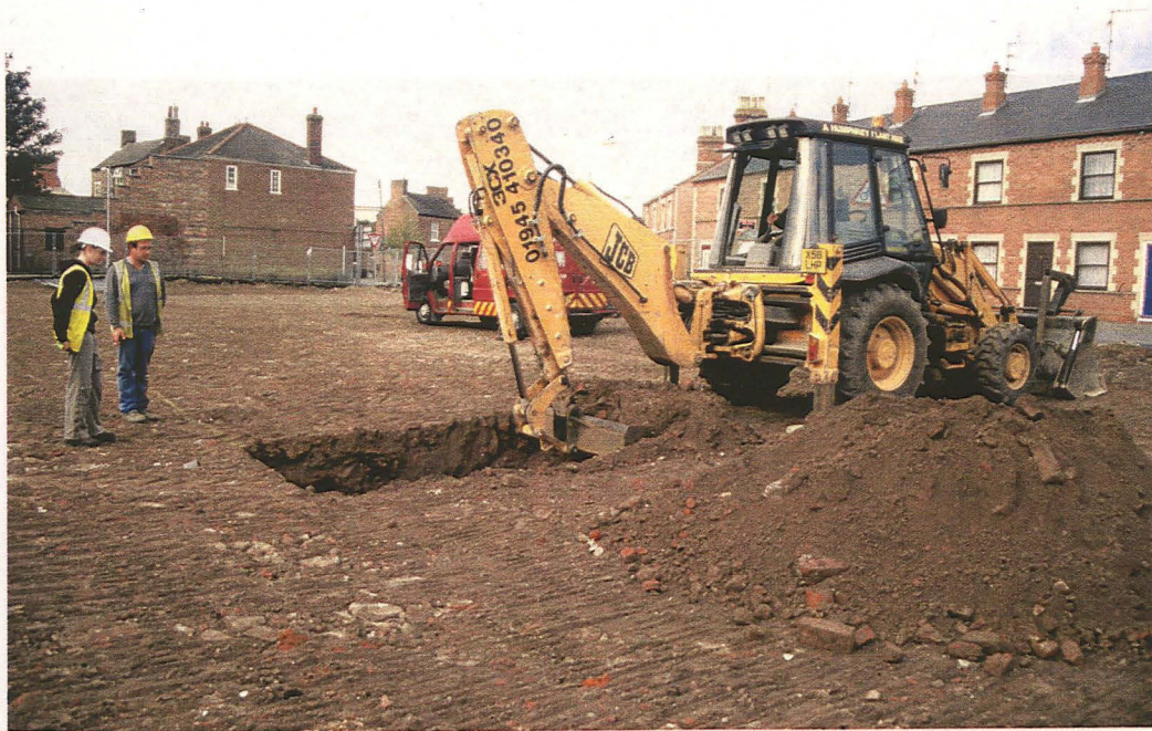
Plate 2 Excavation in progress after clearance and levelling of site.
