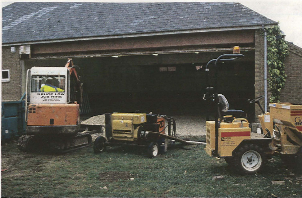
Plate 1 North facing view of site prior to piling
