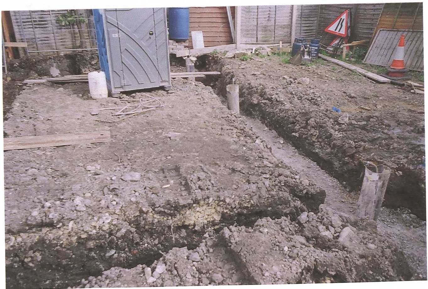
Pl. 8 The site after excavation and partial concreting
