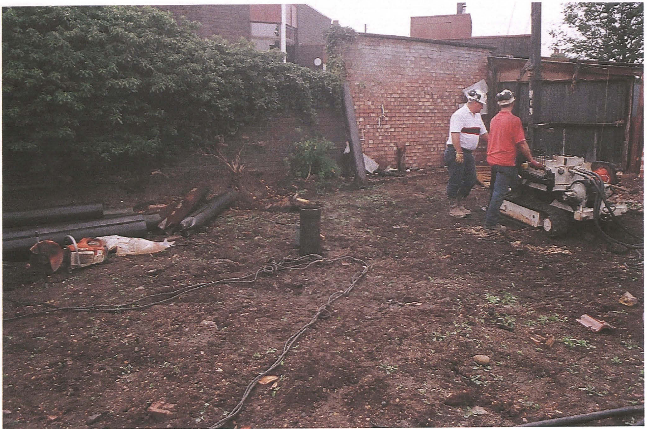
Pl. 3 The piling operation in progress
