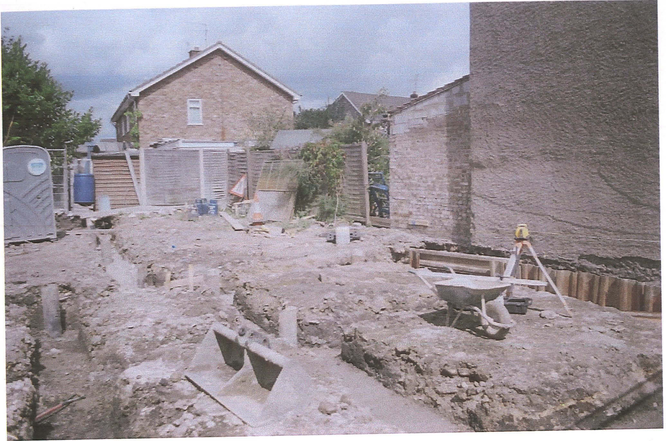
Pl. 9 Looking north-west across completed trenches
