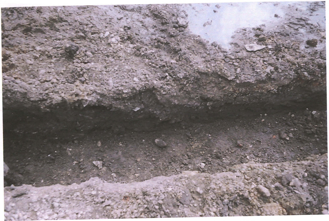
Pl. 7 General view showing typical modern build-up on site and demonstrating the shallow nature of the foundation trenches
