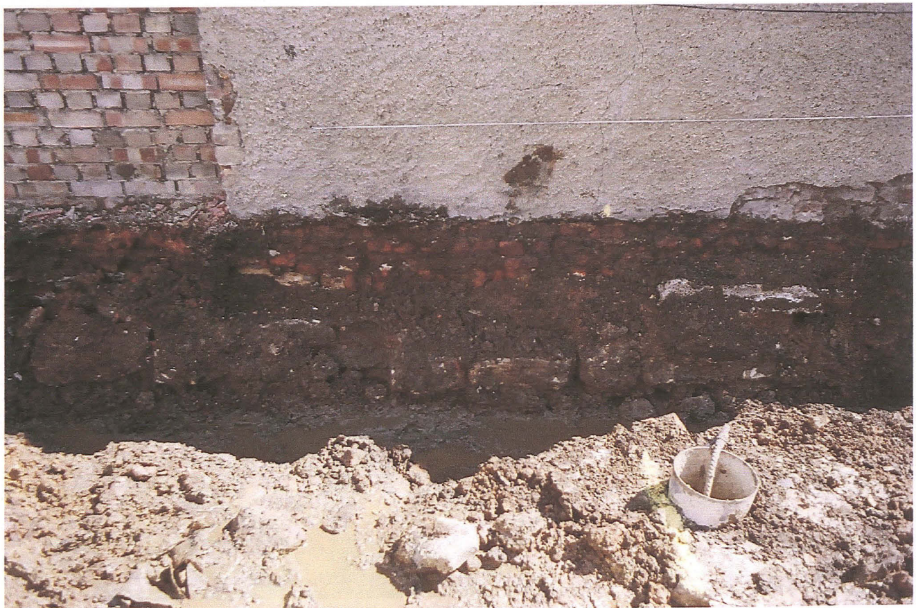
Pl. 4 Exposed foundations beneath 38 East Street showing reused limestone blocks
