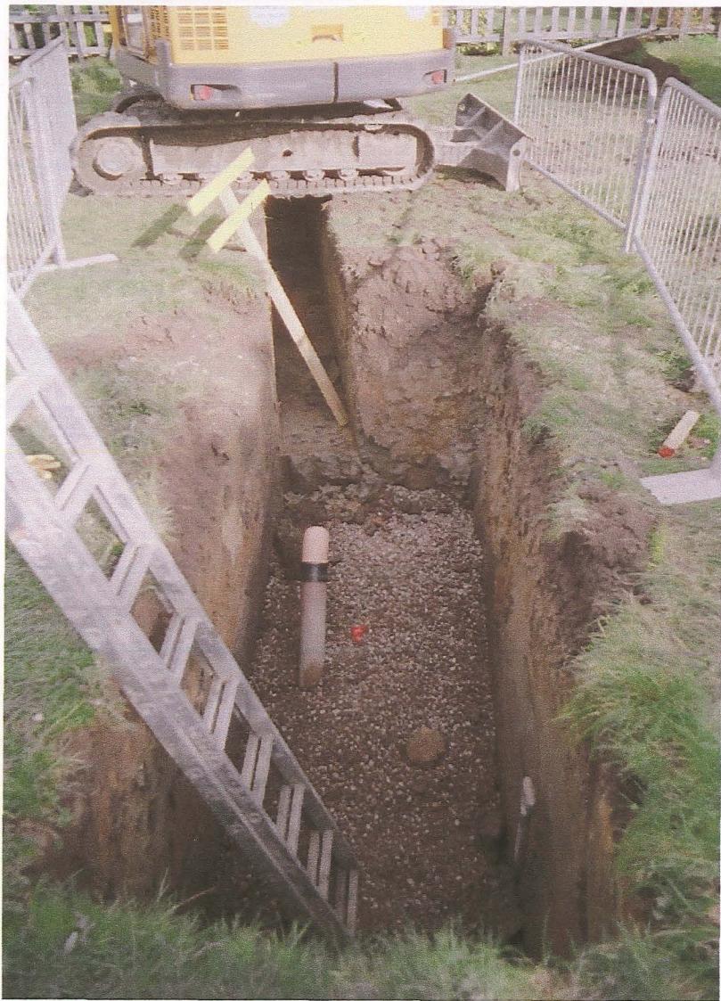
Fig 5. Partially completed pipe linkage leading from the main pipe to properties along the main street
