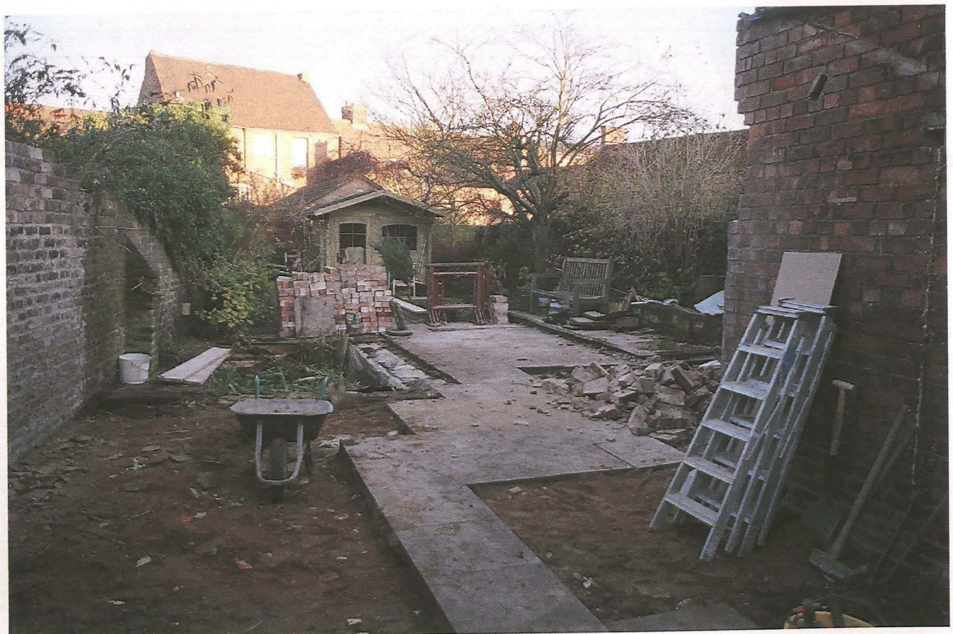
Fig. 2 Looking north across the partially stripped site
