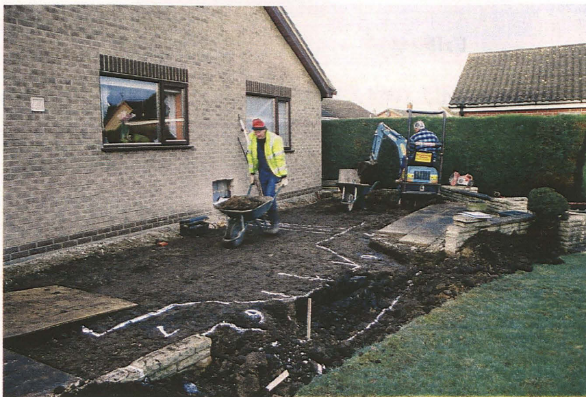
Plate 1 - General view across the development, looking west
