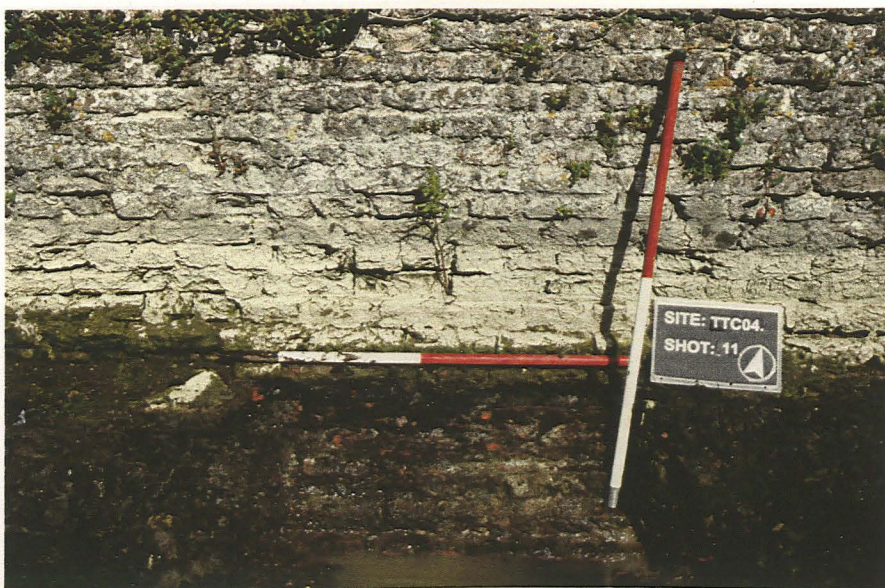
Plate 6 Test Pit 3, looking north.
