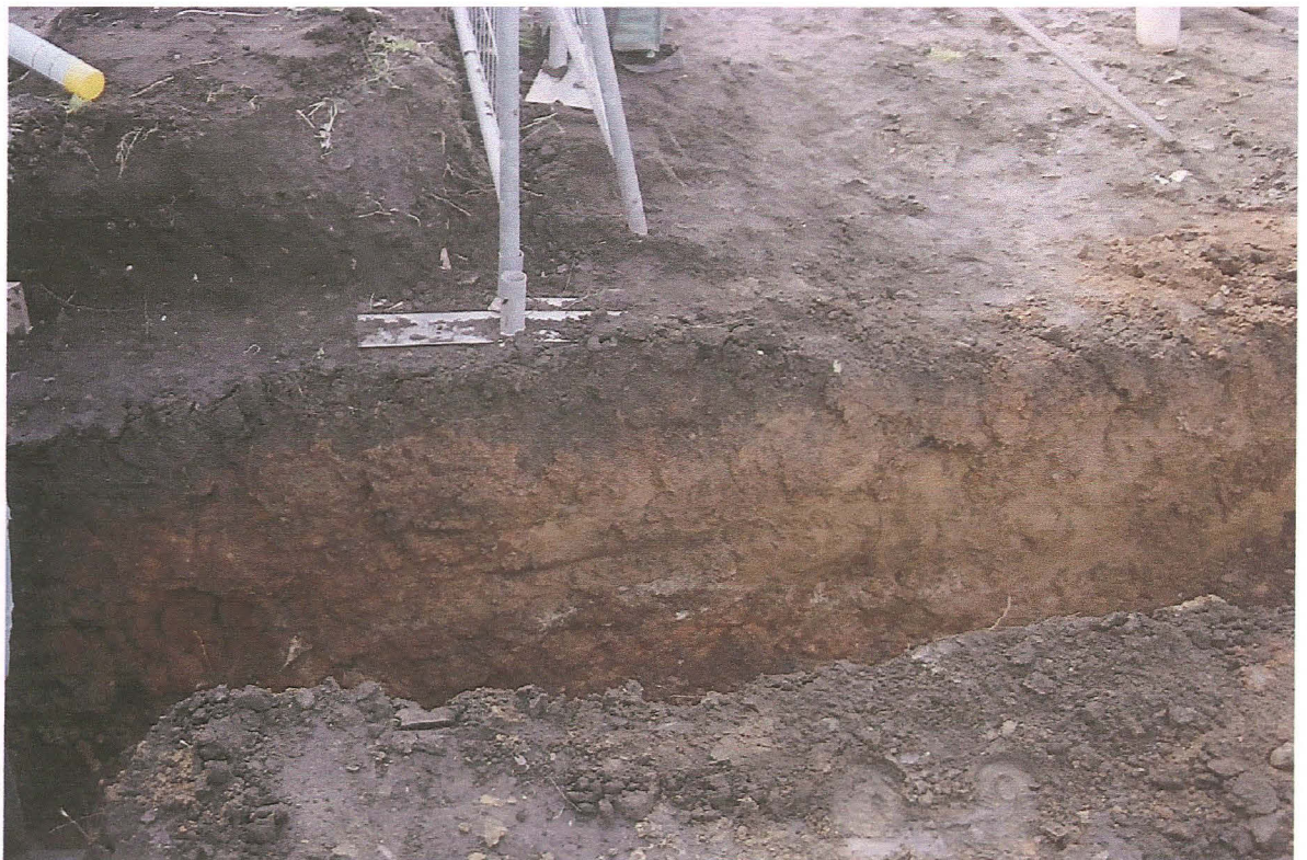
PI. 2 Deposits visible at the eastern end of the southern foundation trench.
