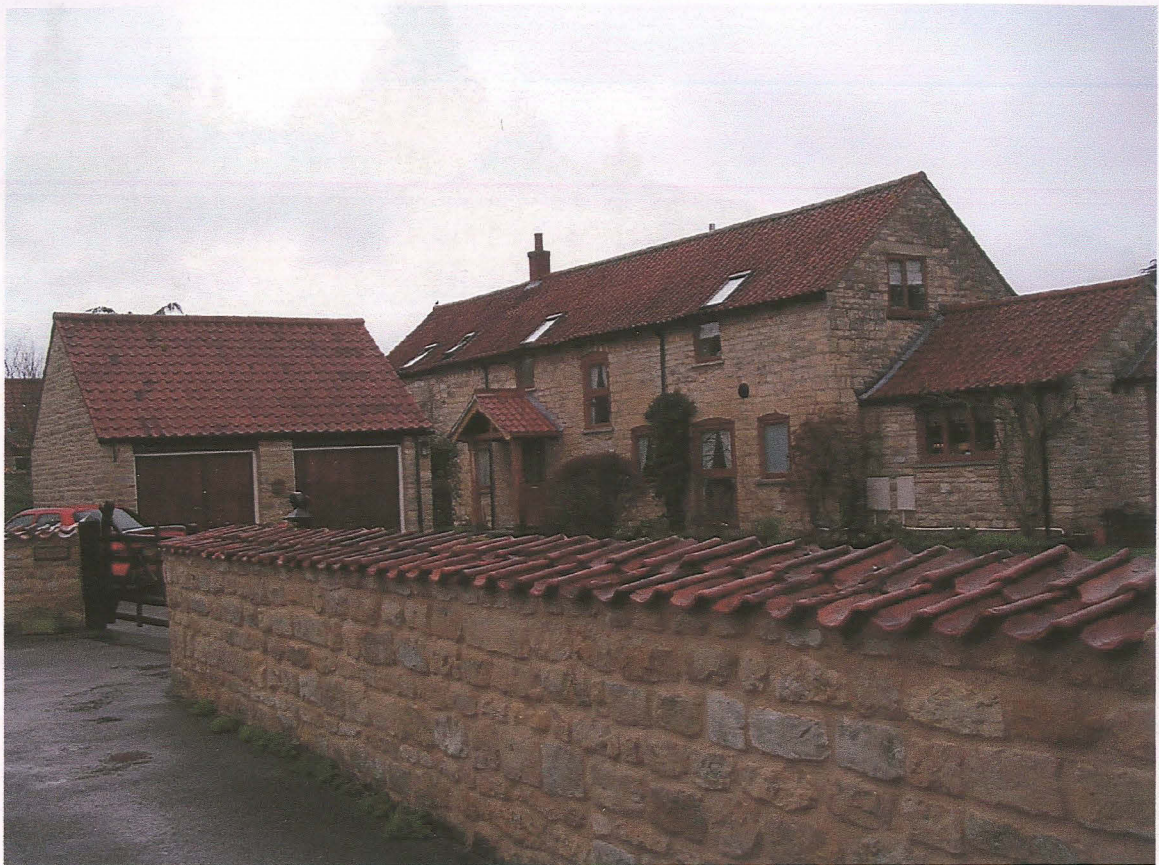
Pl. 7 Converted barn south of Summerdale.
