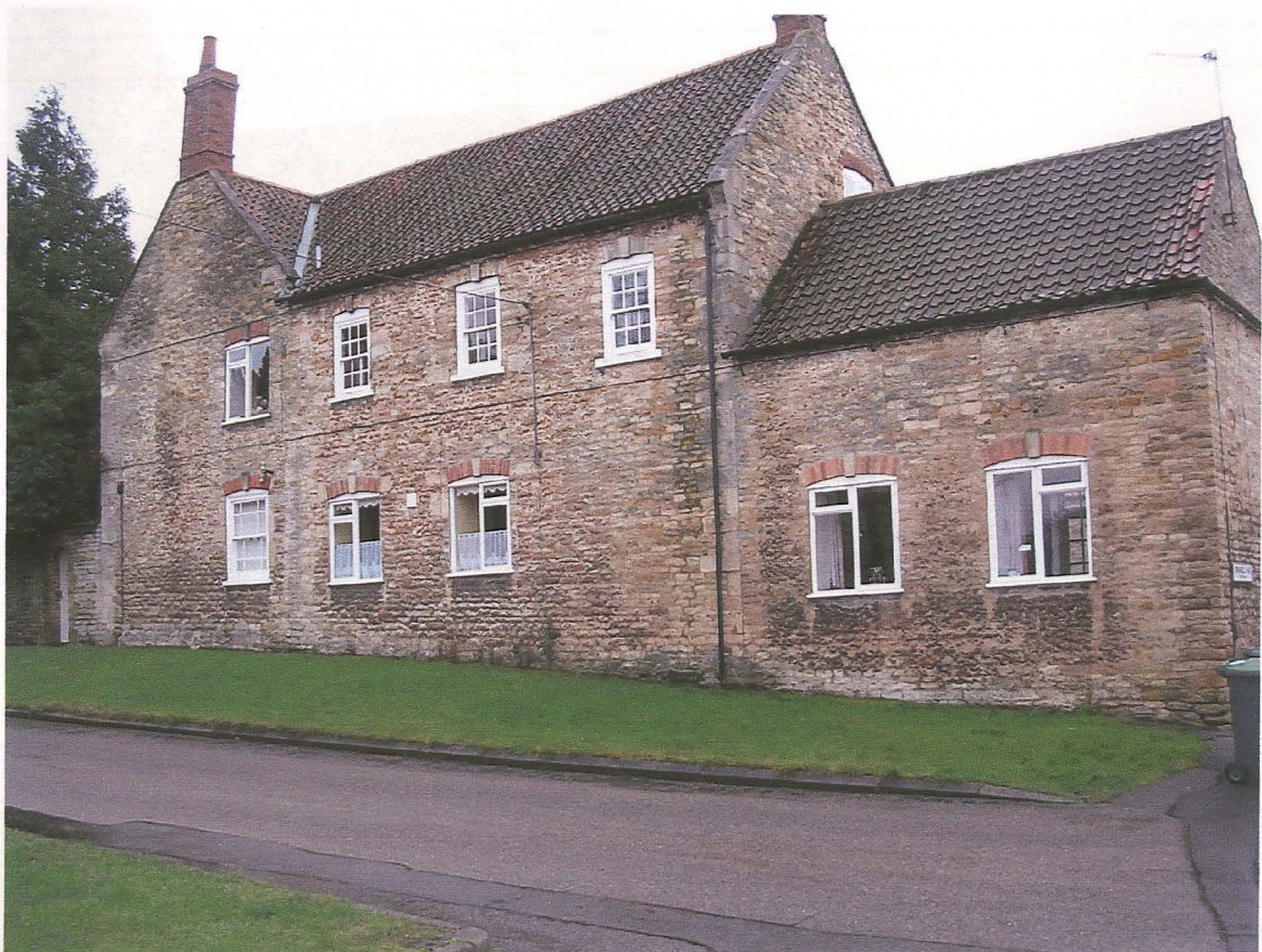
Pl. 2 North elevation of Summerdale, looking south.
