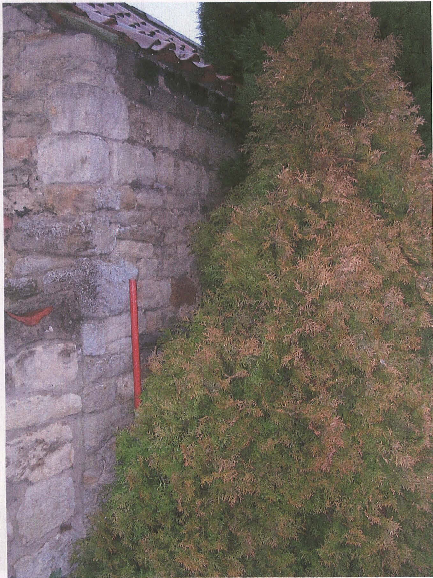
Pl. 11 Blocked entrance in south elevation, to right of 1m scale.
