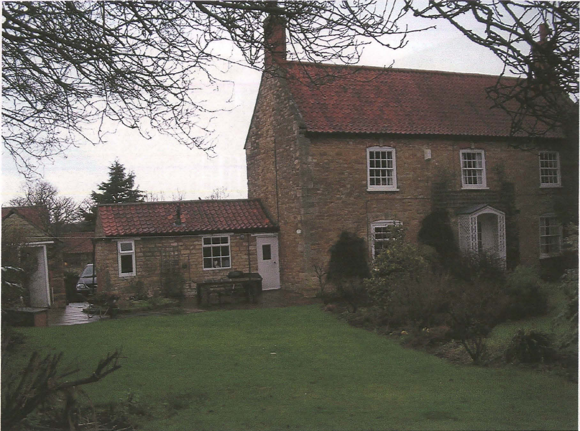
Pl. 1 General view of Summerdale looking west, with outbuilding to left.
