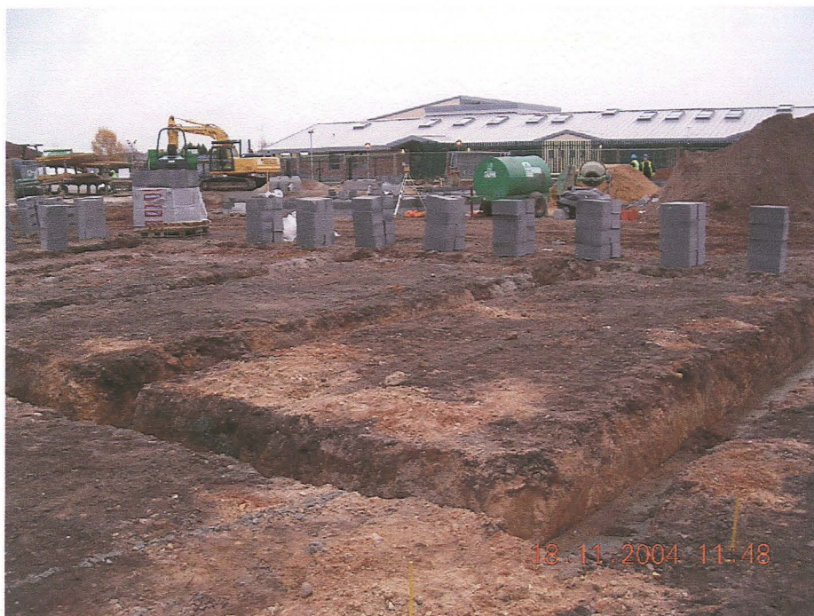
Pl. 4 Very mixed sand deposits were noted across the site and in the house foundation trenches. The variations were interpreted as natural in origin.
