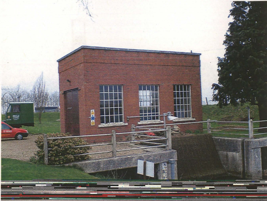
Plate 1 - View showing the position of the proposed sluice/inlet (adjacent to the existing sluice), looking northeast
