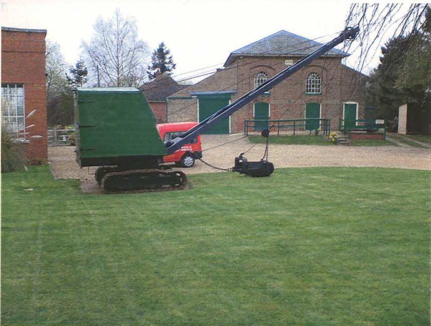
Plate 2 - The proposed site of the new pump house lies beneath the crane and red van. The original 1833 pump house lies in the background, looking southwest
