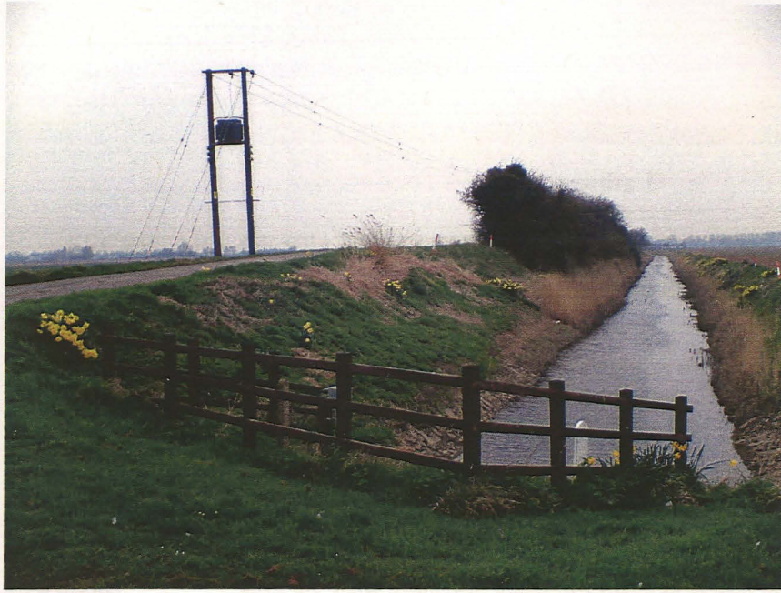
Plate 4 - The Blue Gowt Drain showing the proposed outfall. The medieval sea bank lies to the left and the slight rise in the field surface to the right indicates the position of a medieval saltern, looking north
