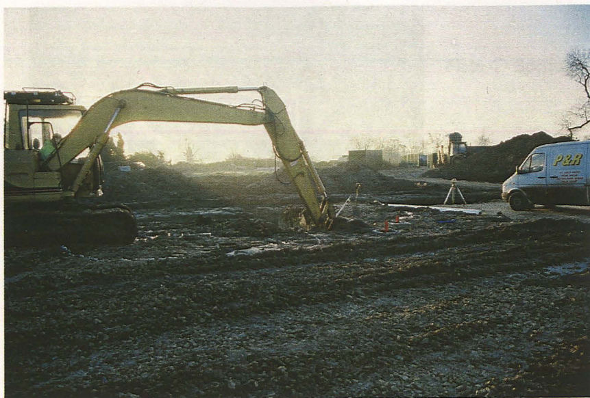
Plate 1 - View across Plot 1, looking south
