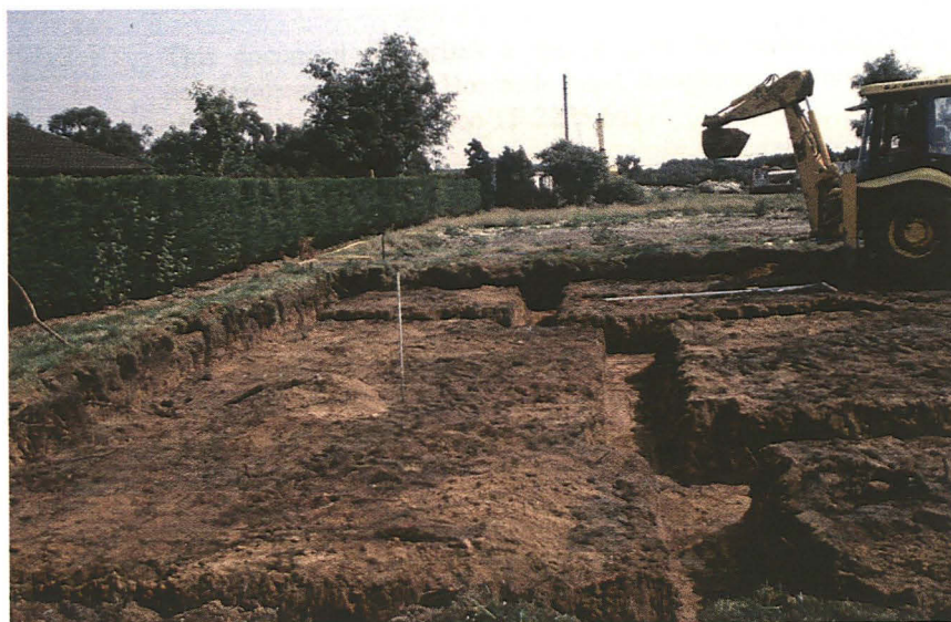
Plate 5 - Excavated foundation trenches Plot 11, looking northwest
