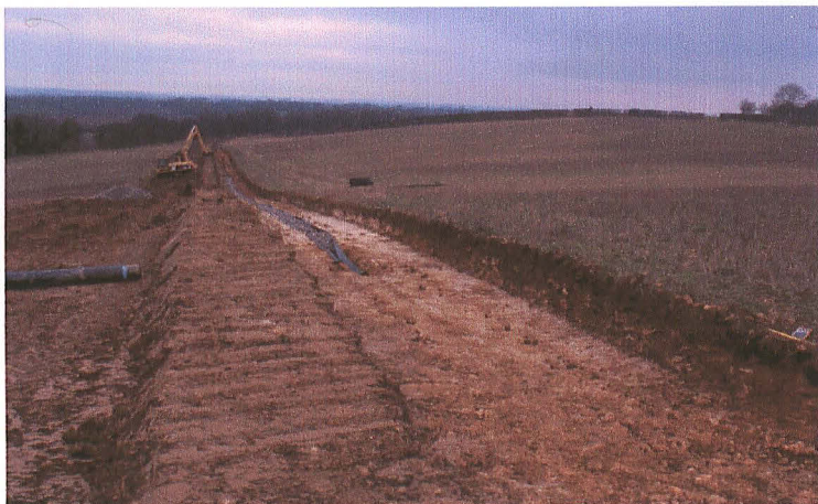
Pl. 7: View along line of gallop, north westwards from southern end.
