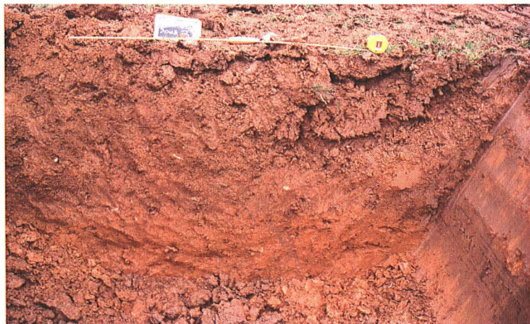
Pl. 3: Section from soakaway 3. Looking West.
