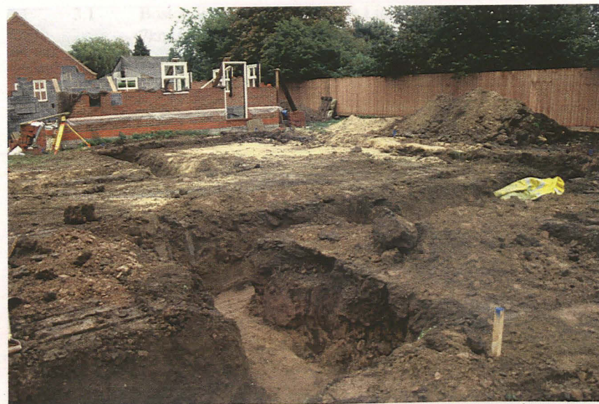
Plate 10 - Plots 4/5: Showing excavation of foundation trenches, looking south
