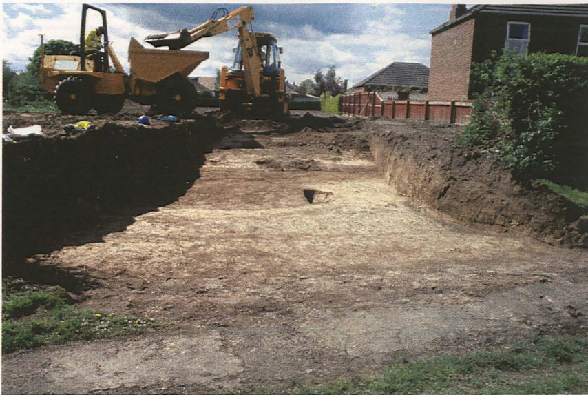
Plate 1 - View showing the stripped Access Road, looking west
