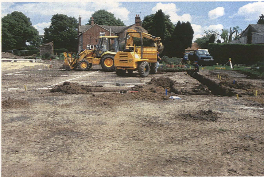
Plate 7 - Plot 2: Excavation of foundation trenches, looking east
