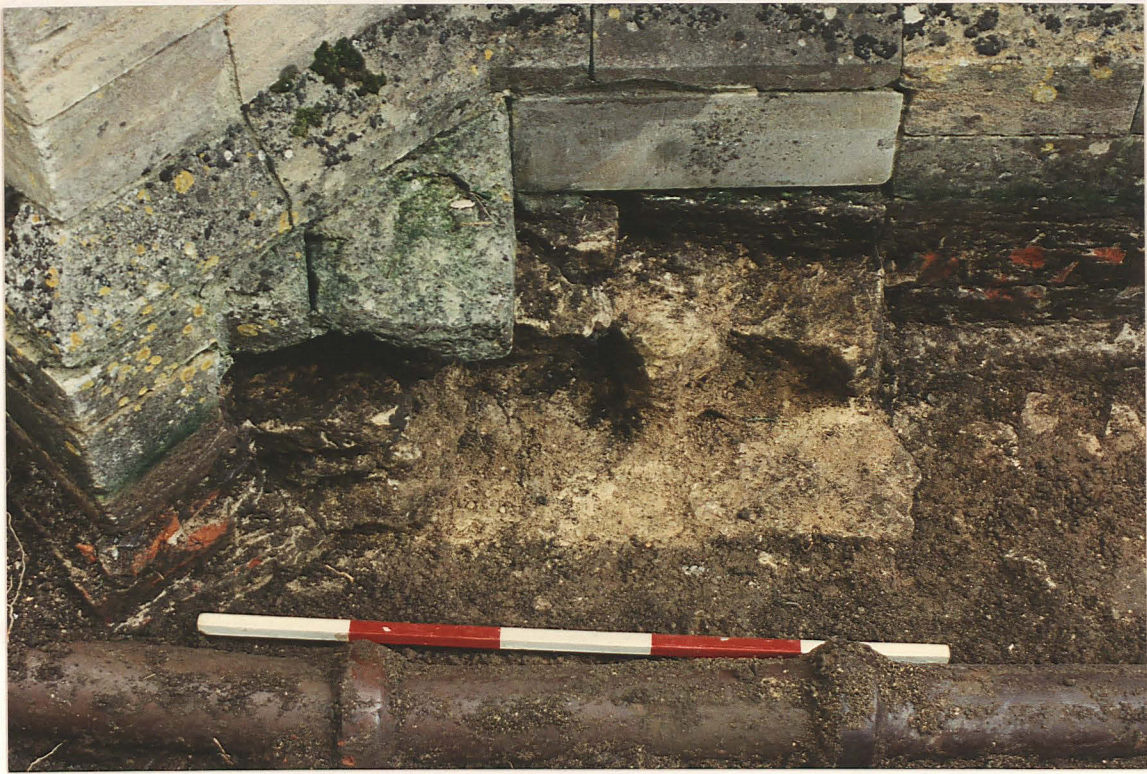
Pl. 29. Close-up of clasp buttress foundations in N aisle N wall.
