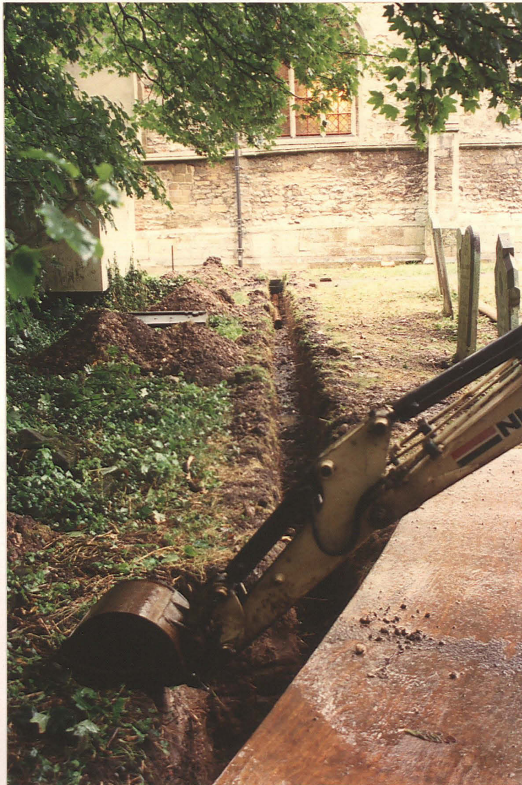
PI. 46. Soakaway trench running S of church.
