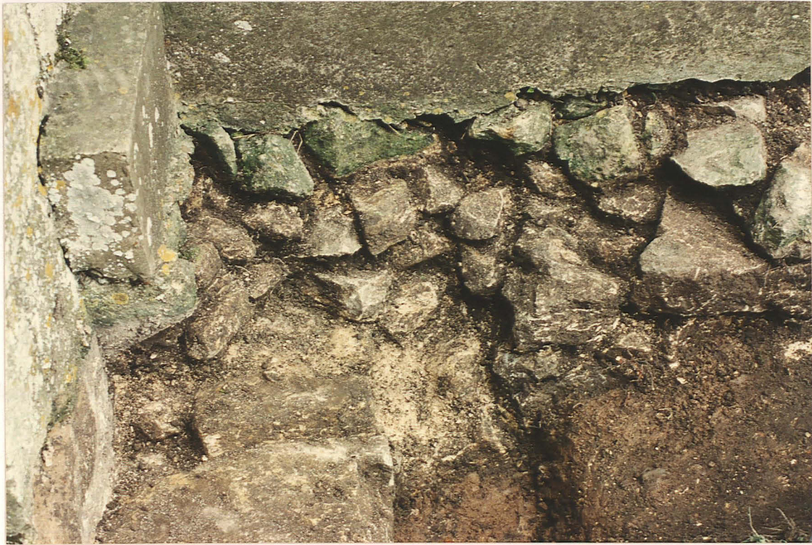
Pl. 37. Rubble packing (10) above (11) overlying nave foundations.
