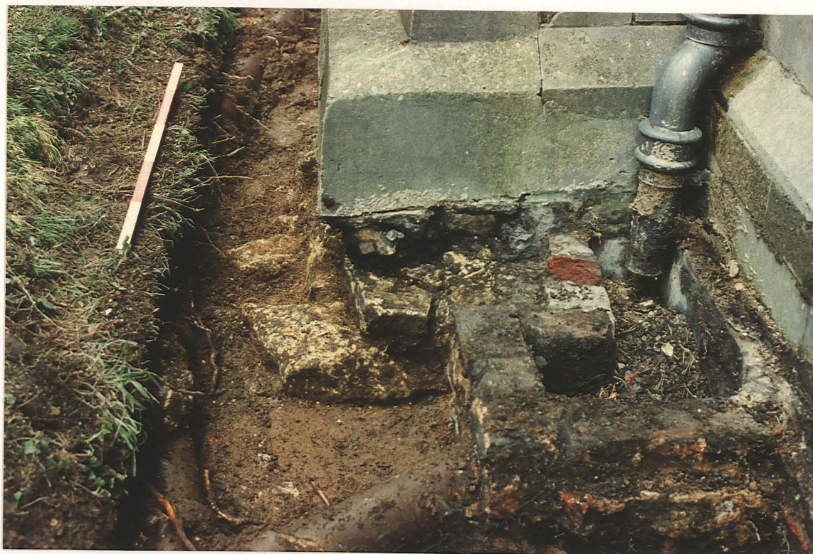
Pl. 32. Foundations beneath buttress in N aisle (8) W side.
