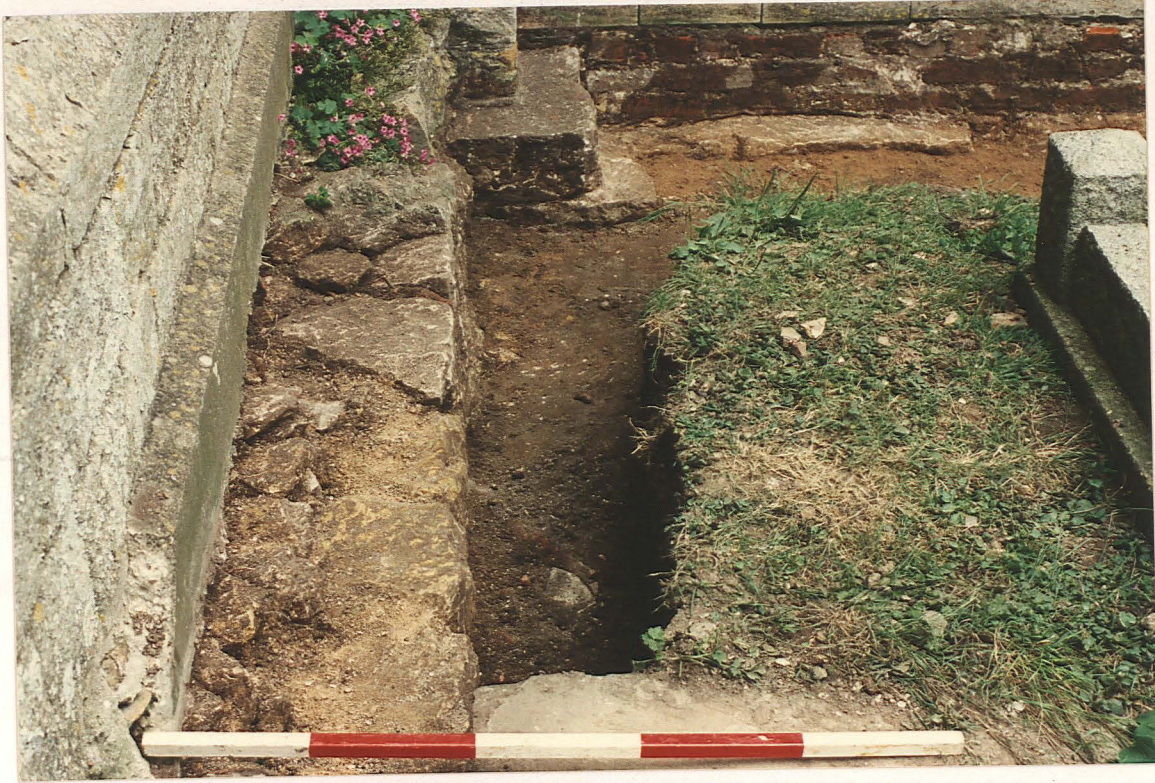
Pl. 41. Stone foundations to S of nave. Remains of 13th century S aisle.
