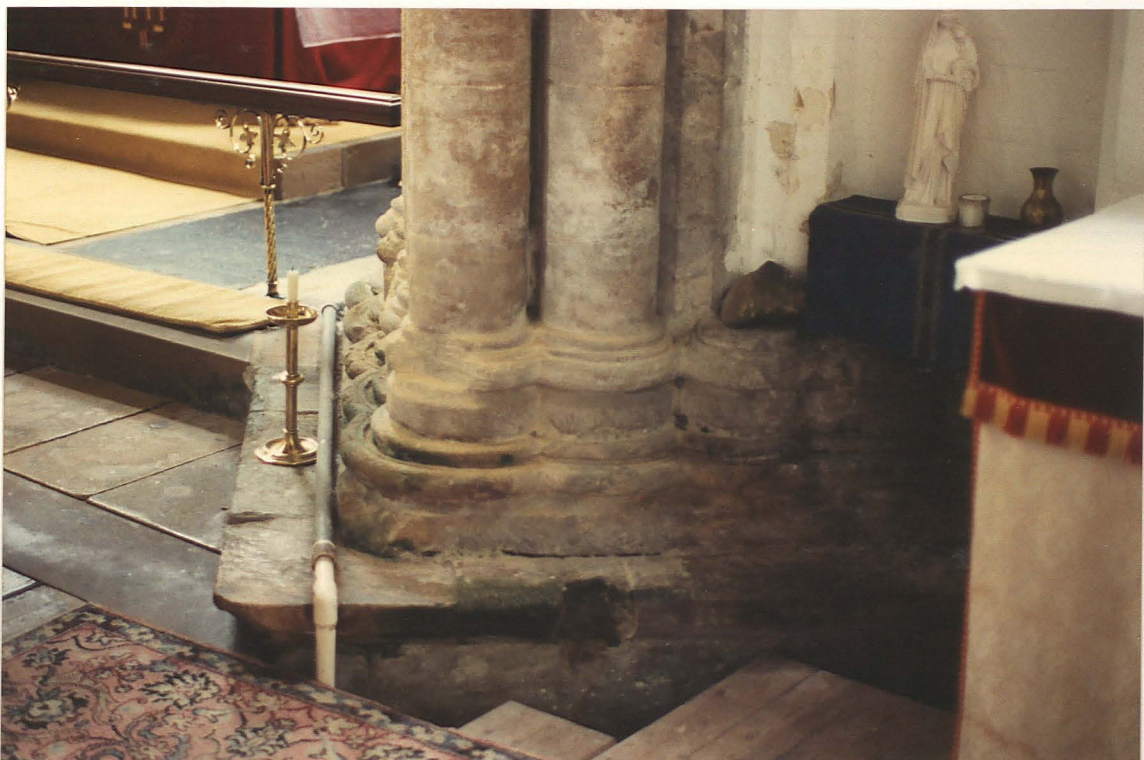
Pl. 6. SE pillar of central tower crossing (now the S pier of the chancel arch).
