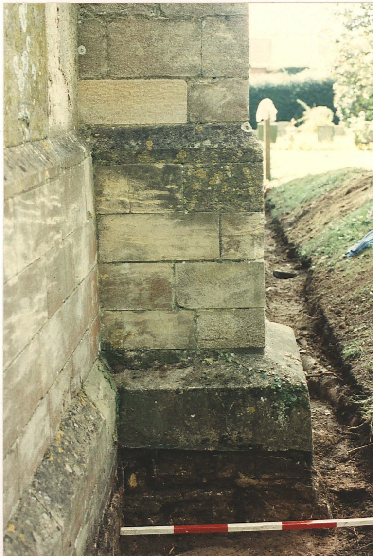
Pl. 30. Foundations beneath buttress in N aisle (8) E side.
