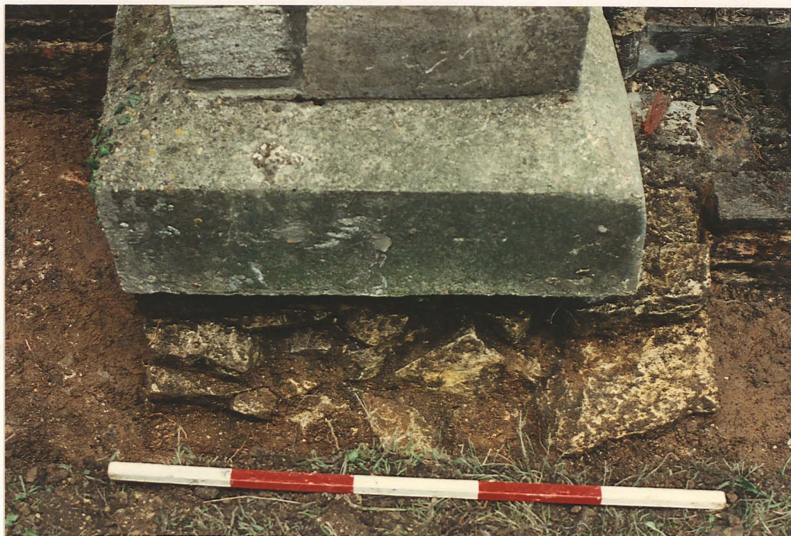
Pl. 31. Foundations beneath buttress in N aisle (8) N side.
