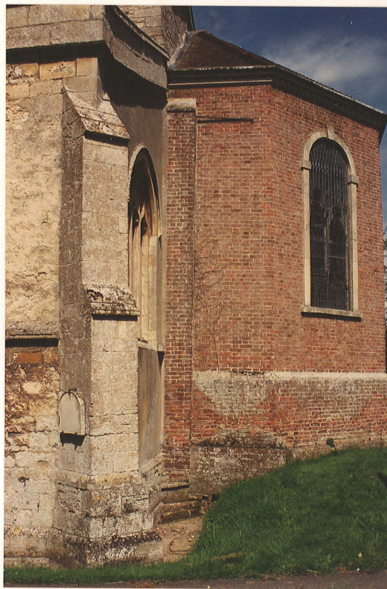
Pl. 17. Apse SE angle showing remains of setting out course. (looking E).
