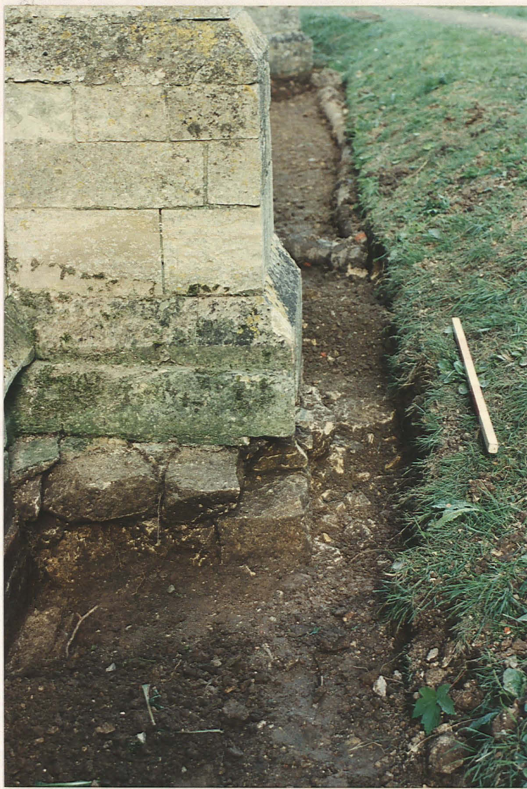
Pl. 43. Foundations beneath S aisle buttress marking position of earlier S transept (W side).
