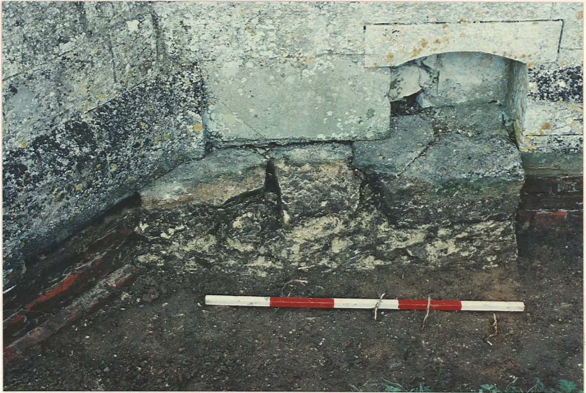
Pl. 23. Close-up of door jamb leading to S chapel (built over by later aisle buttress to L).
