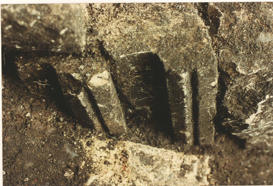
Pl. 36. Re-used window jambs in underpinning beneath tower N wall.
