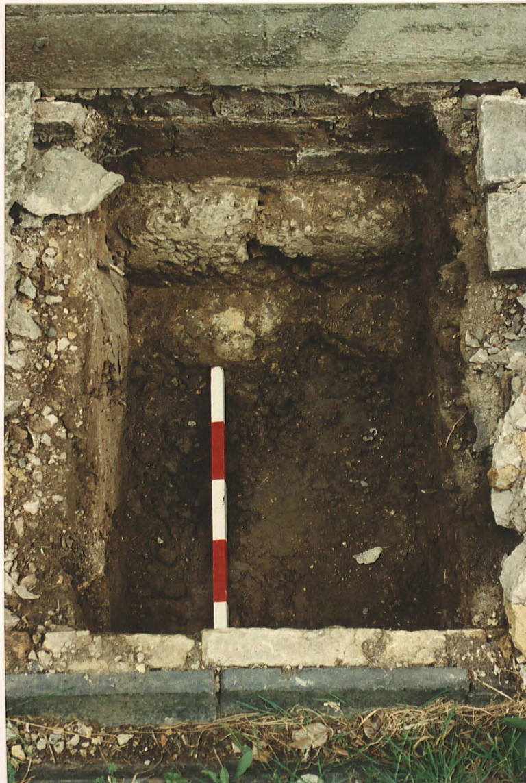
Pl. 13. Test pit 2 showing brick and concrete underpinning.
