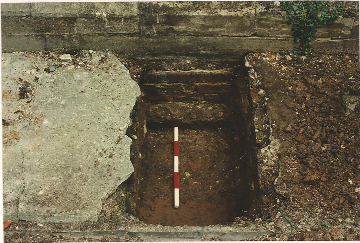
Pl. 9. Test pit 1 showing brick and concrete underpinning. (Scale 0.50m)
