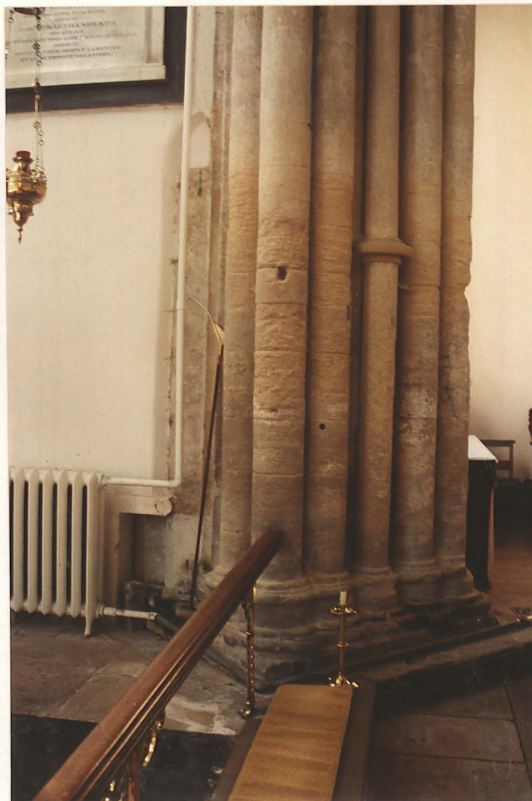
PI. 19. Junction of apse and S aisle showing cushion base and tablet.
