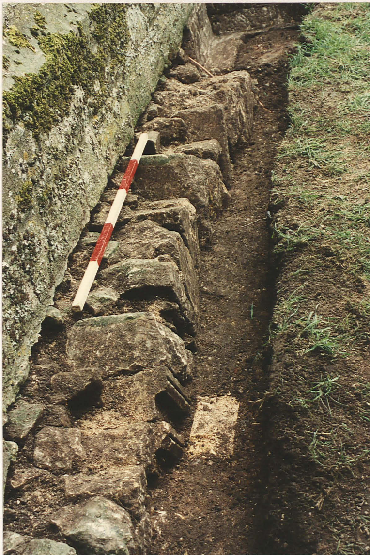
Pl. 35. Underpinning (11) beneath tower N wall.
