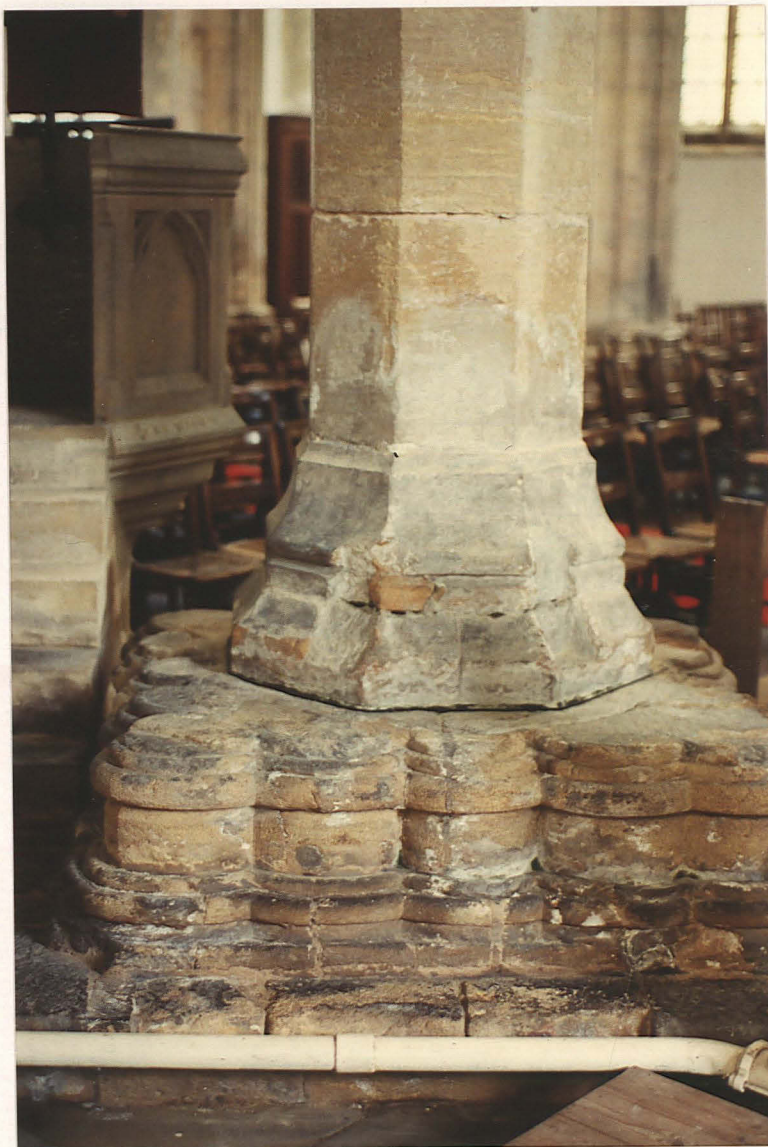
Pl. 7. SW pillar base of central tower crossing, re-used to support 15th century aisle pillar.
