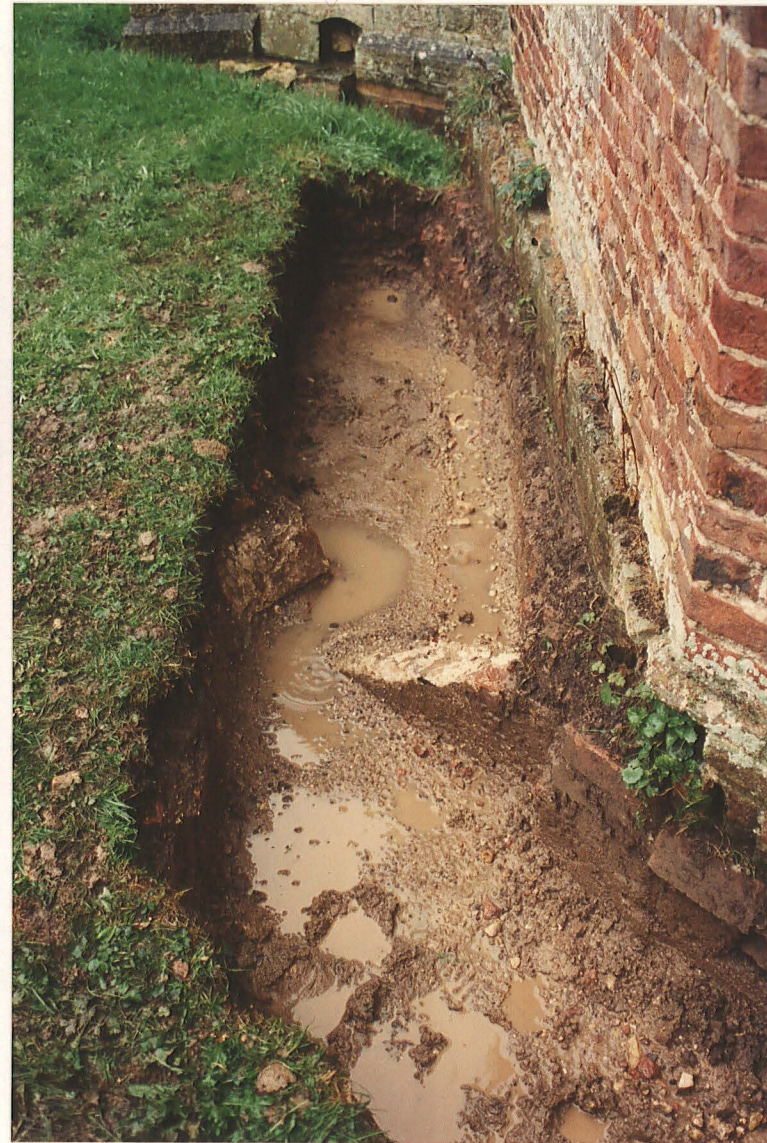
PI. 15. Apse E wall showing shallow foundations.
