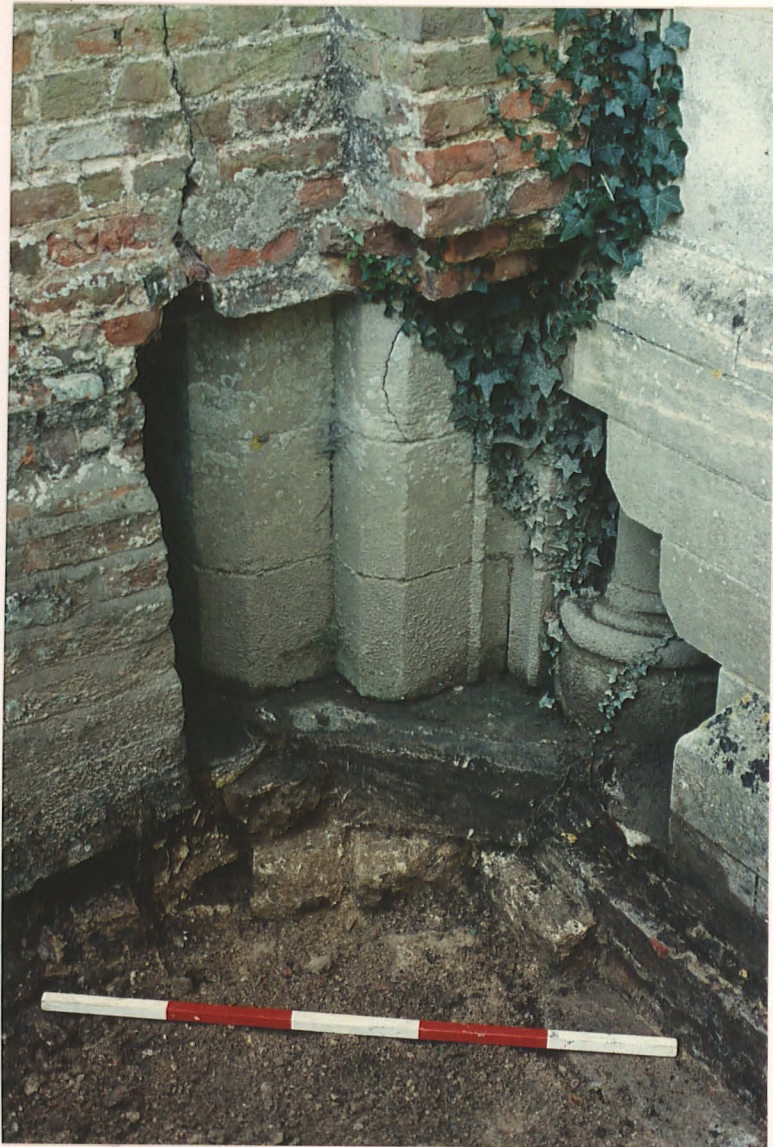
Pl. 25. Junction of apse and N aisle showing arch/door jamb for access between chancel and the N chapel (L) and cushion base (R).
