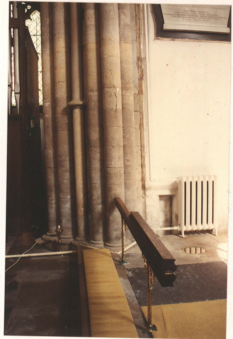
Pl. 25. Junction of apse and N aisle showing arch/door jamb for access between chancel and the N chapel (L) and cushion base (R).
