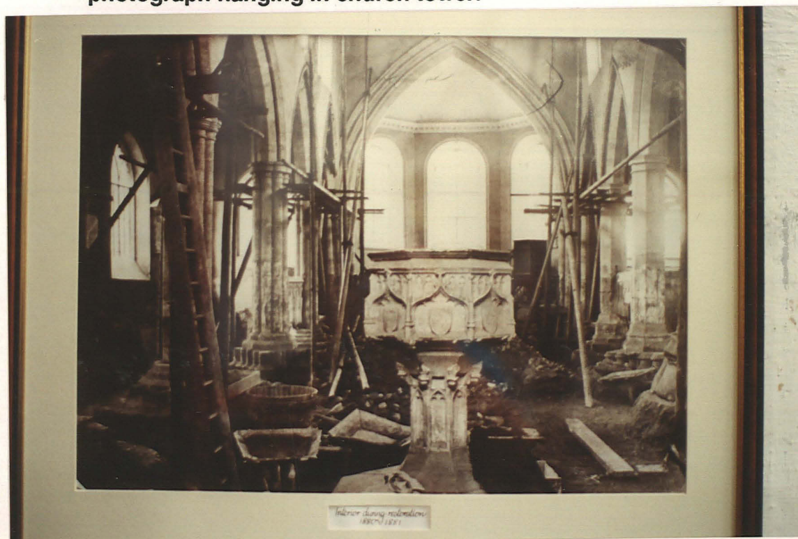
Pl. 8. Church interior looking towards apse in 1881 during repair work. Note central window in apse (now blocked). Copy of photograph hanging in church tower.
