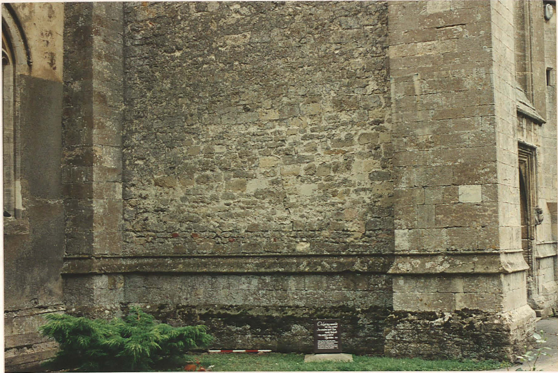
Pl. 33. Tower N wall showing buttress at angle with N aisle.
