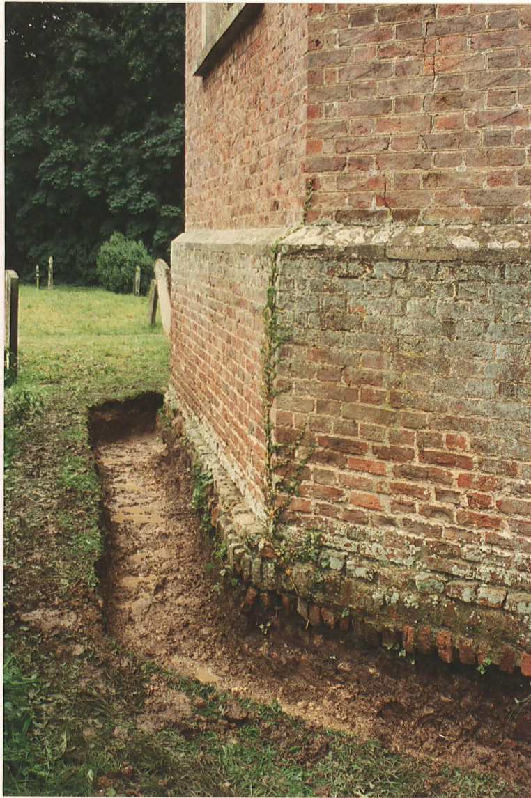
PI. 15. Apse E wall showing shallow foundations.
