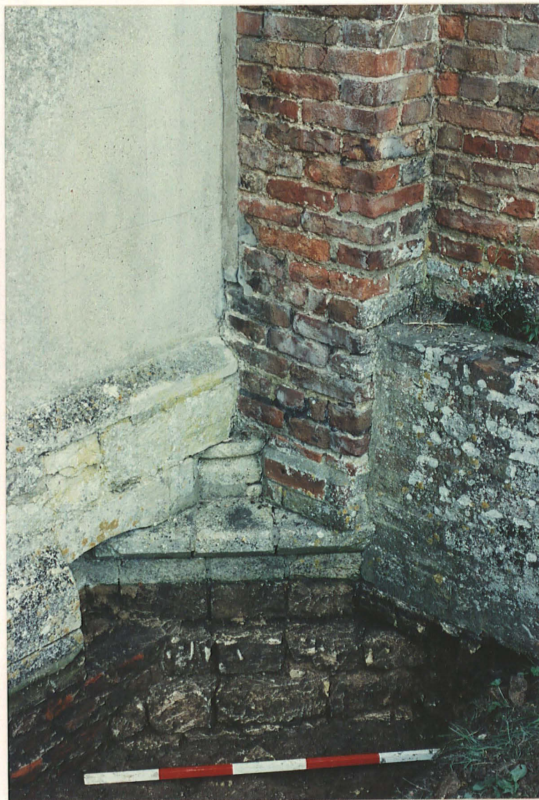
PI. 19. Junction of apse and S aisle showing cushion base and tablet.
