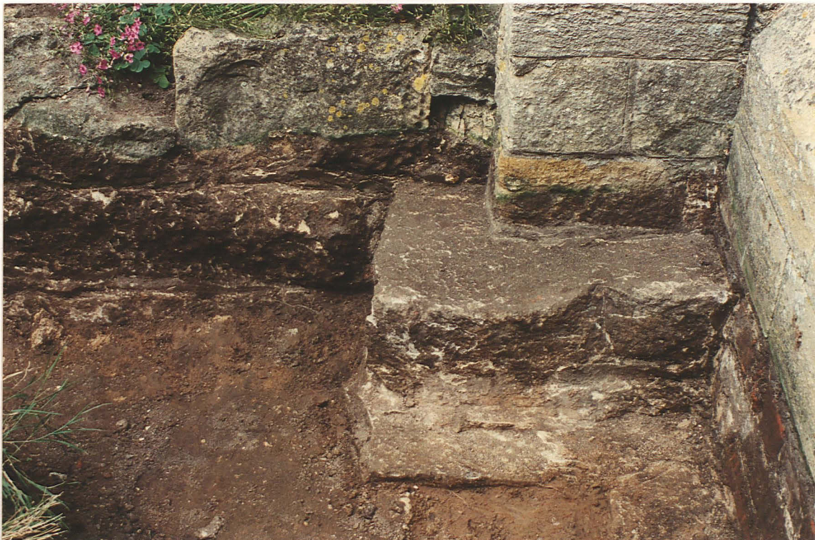
PI. 40. Nave foundation beneath later buttress at angle between tower S wall and S aisle.
