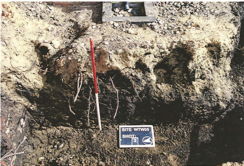
Plate 2 - Section 1 showing the general sequence of deposits in the foundation trenches for the new extension, looking east
