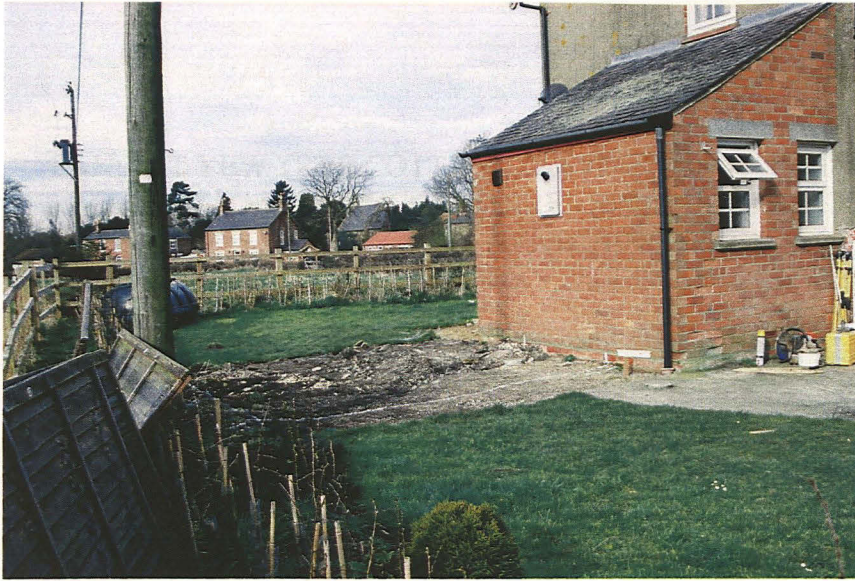
Plate 1 - View showing the area of extensions prior to excavation, looking northwest
