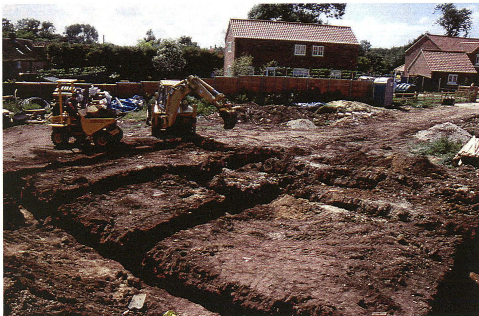
Plate 2 View of Plot 5 during excavation
