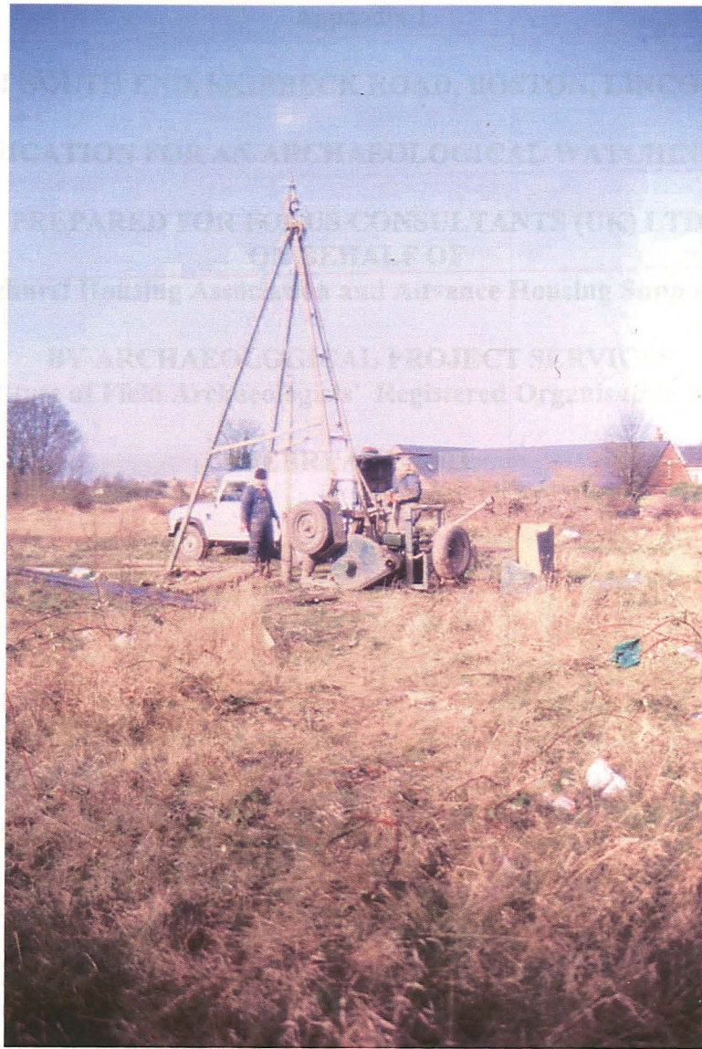
Plate 1 General east facing view across site showing boring in progress
