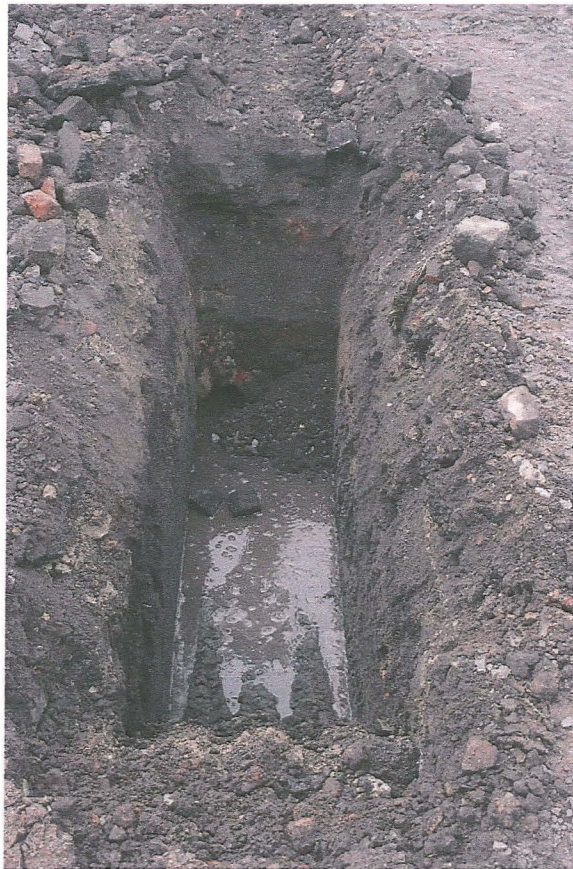
PI. 16 Part of a brick culvert 650 and a brick wall 649 were seen at the southern end of Trench J (looking south).
