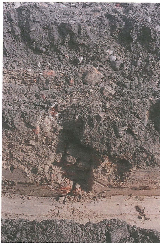
PI. 14 Brick wall foundation 643, in the northern face of Trial Pit E. This may be part of Mr Keyworth's house.
