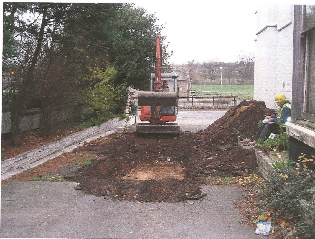
Pl. 1 21 – 25 St Catherines, Lincoln, trench location view looking east.
