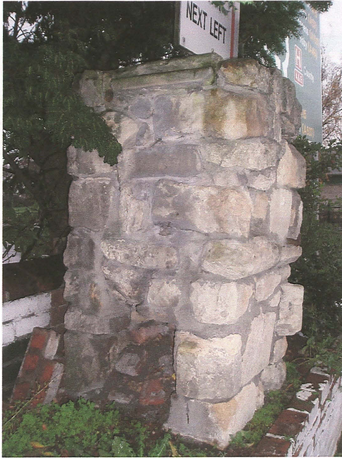
Pl. 11 Pier in front garden of 21 St Catherines incorporating re-used masonry.
