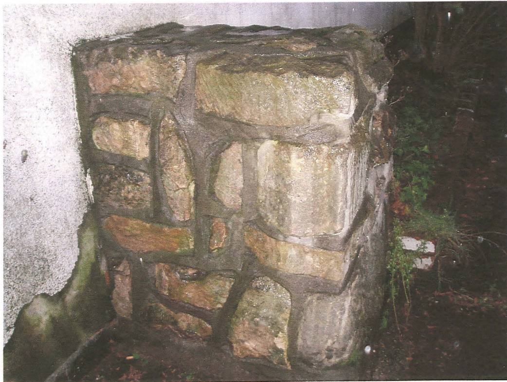
Pl. 14 Pier 2 at rear of 21 St Catherines incorporating re-used masonry. West face.
