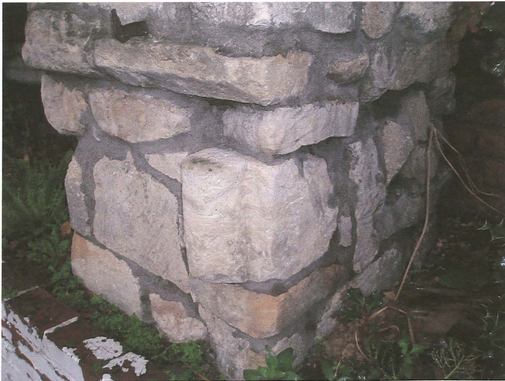
Pl. 12 Detail of pier showing chamfered blocks on south face.
