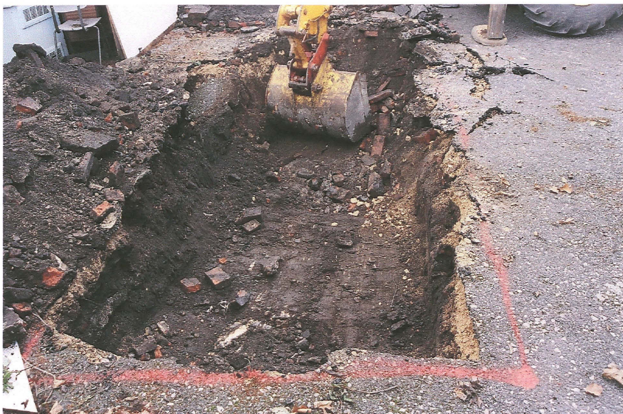
Pl. 3: Trench 1 under excavation, facing east.
