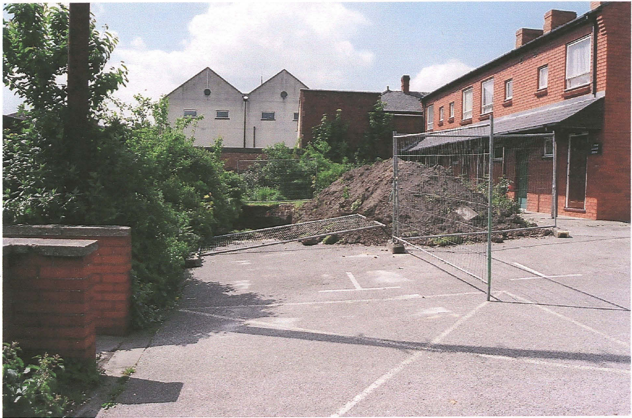
Pl. 5: General site shot showing Trench 2 in the garden, facing west.
