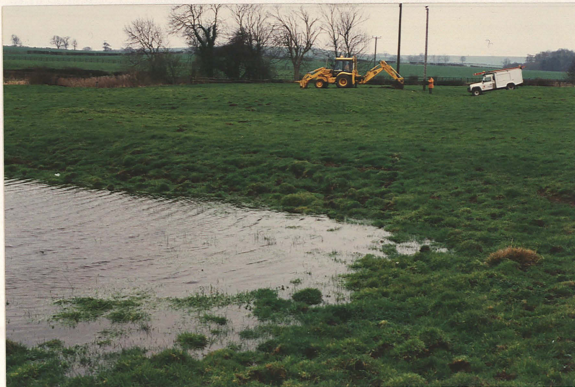
Pl. 23 Location of Hole 16 on ridge to south of Calceby fishponds, looking south
