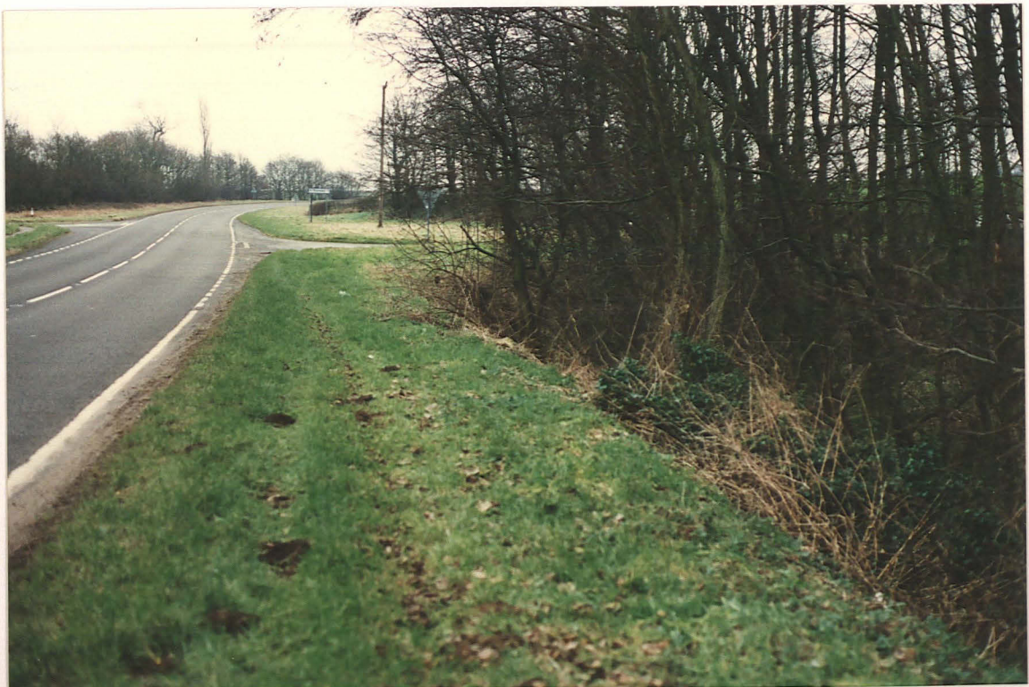
Pl. 13 Realigned road junction of A16 and the Calceby road, with trees to right growing in lower ground (facing east)
