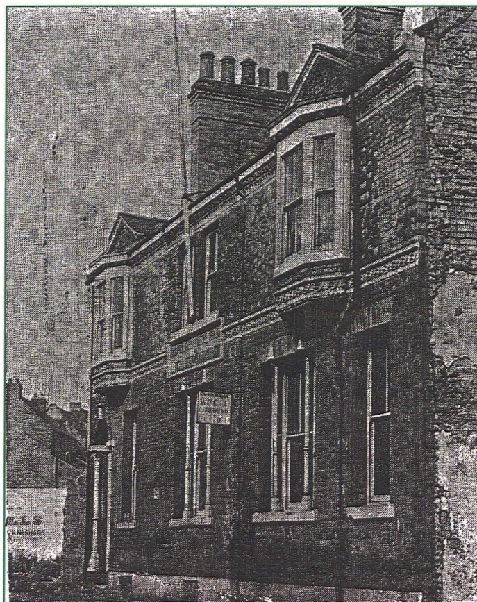
Plate 1 (above): The 19 th century Working Men's Club at nos. 19-21, Bridge Street, awaiting demolition in 1976. Note the rough brickwork of the near gable end, showing that an abutting building has already been demolished.
