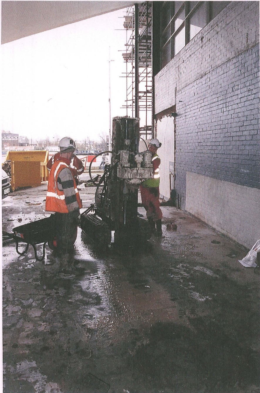
PL. 3 The piling rig in operation
