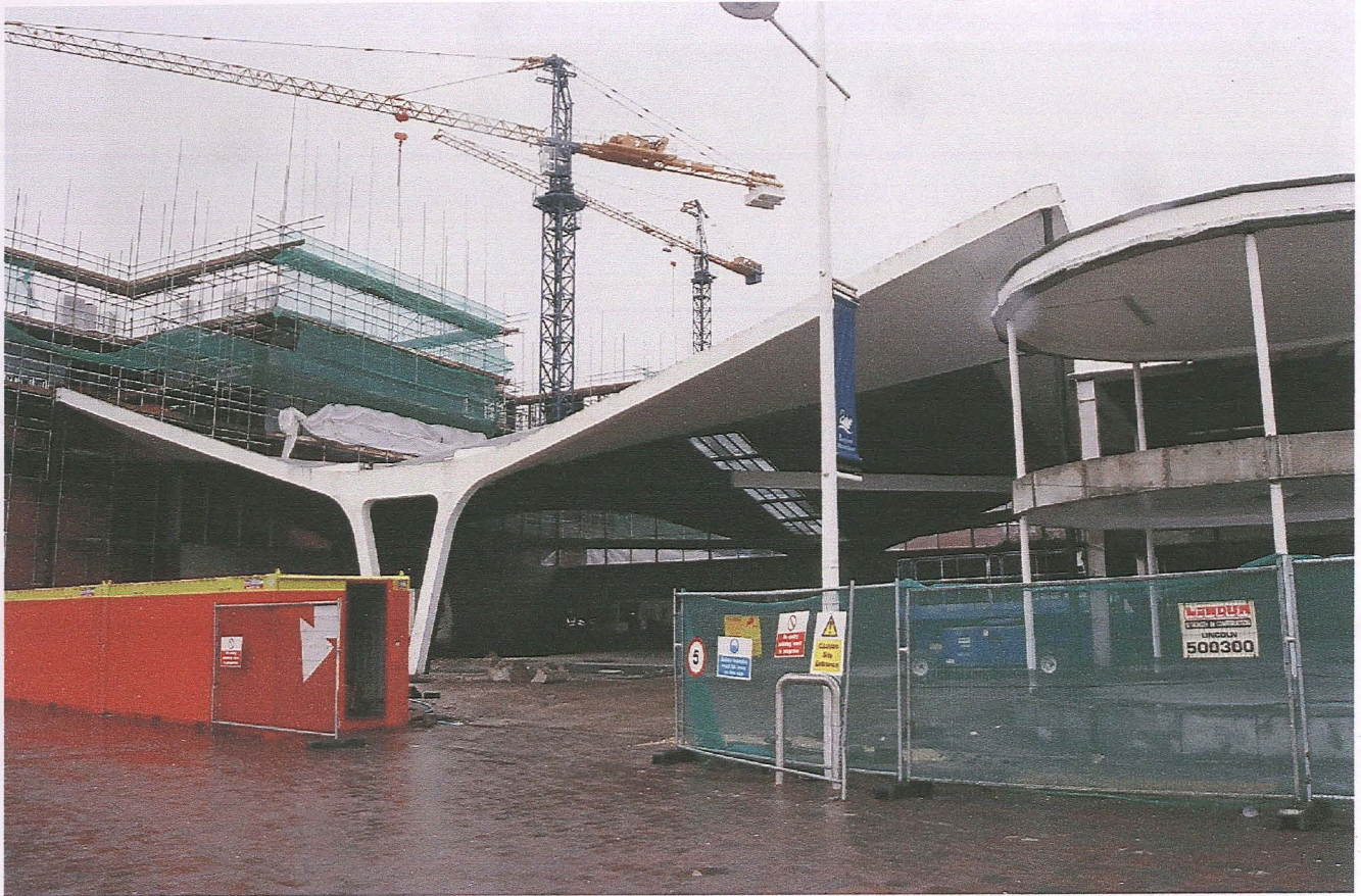
Pl. 1 Exterior view of the development prior to piling operations
