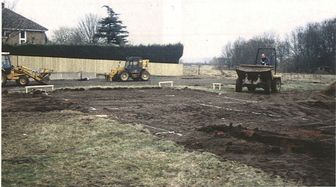
Plate 1 General view of site
