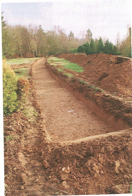
Pl 6 Trench 2 cleaned looking south-east Scales 1m and 2m
