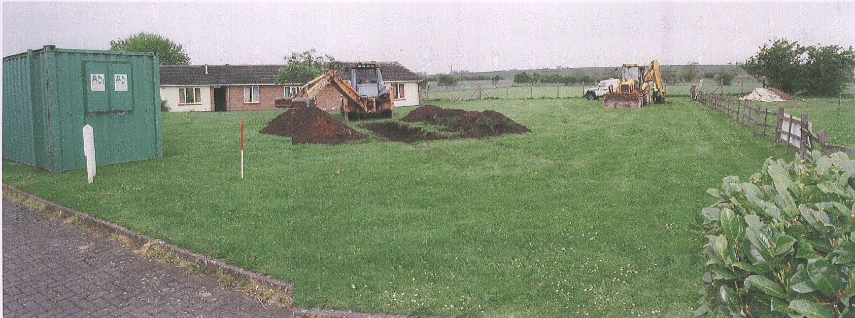
Pl. 1 Area 1, general view looking west
