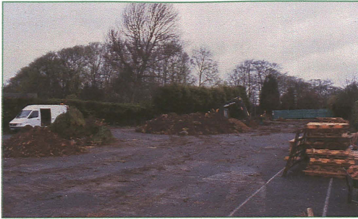
Plate 1. General view of the development area, looking North-East
