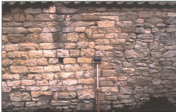
Pl. 5: Detail of scar at east end of wall. To the west is a possible putlog hole. Looking north.
