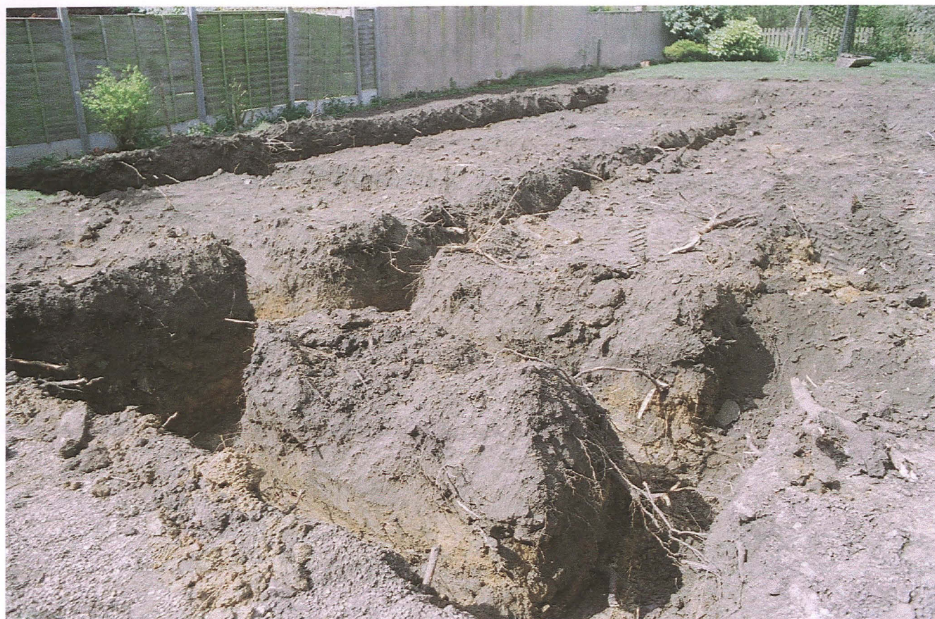
Pl. 5 Looking north-east across the excavated foundations showing root damage in the foreground
