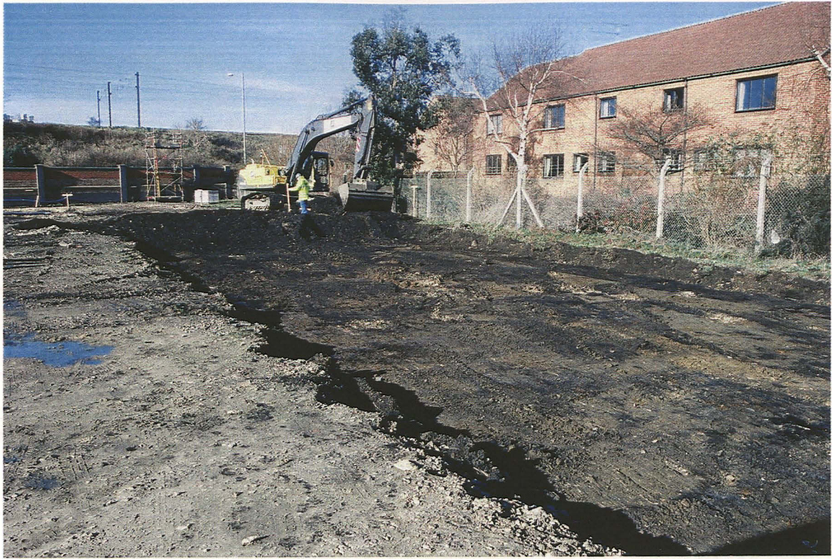
Plate 1 Stripped area at north end of site, looking north-west
