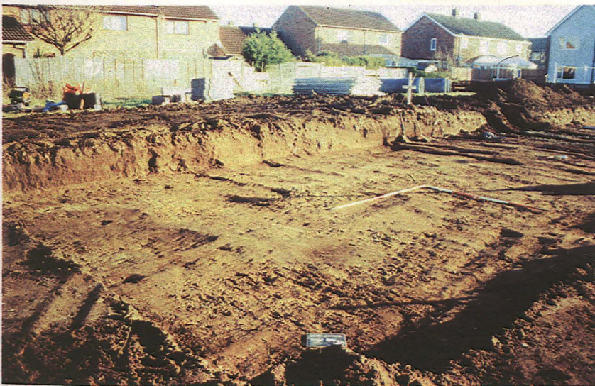
Plate 24 South facing view of road strip at northern end of Road 2.
