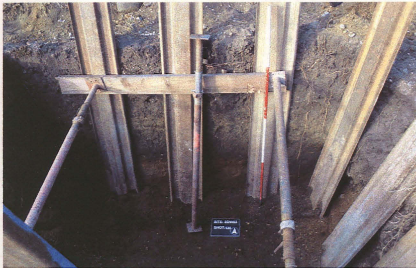
Plate 17 South facing section Manhole 1 (MH1) (Section 54).
