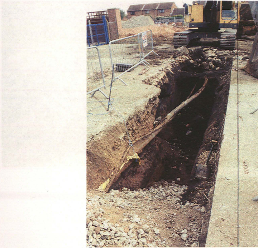
Plate 16 East facing view of service trench FW05-MH1 during excavation.
