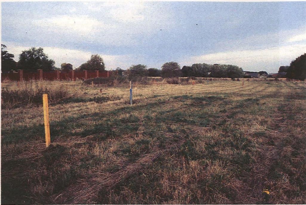
Plate 1 North facing view of development area prior to the commencement of excavation.
