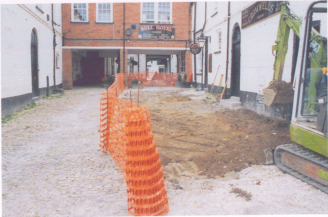
Pl. 1 View of courtyard, looking west, during removal of existing surface.
