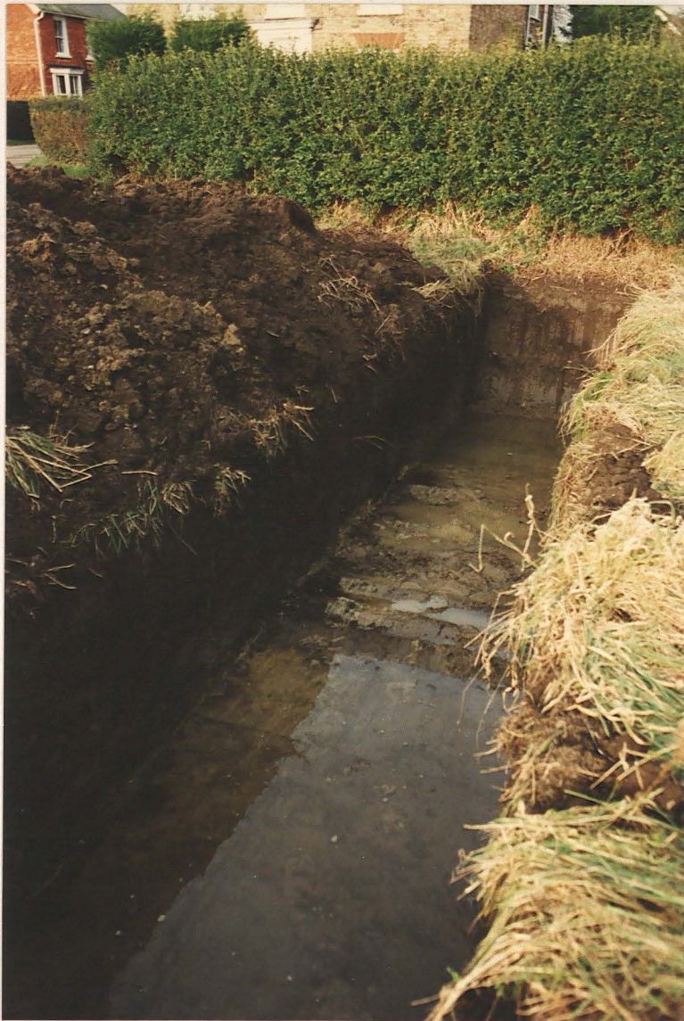
Pl. 3 Hagnaby Lane trench, view N. Same view as Pl. 2 after 3 hours, showing water seepage.
