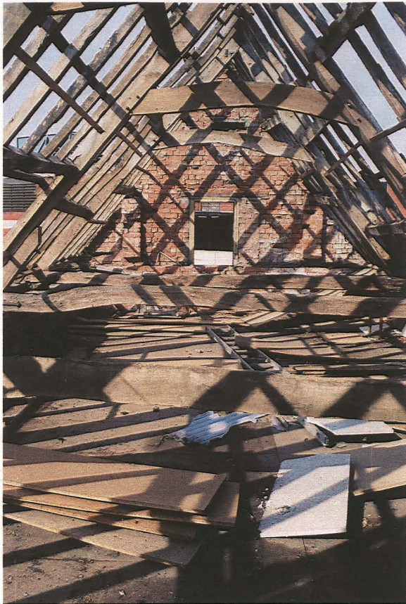
Plate 3 Interior of attic, showing partially blocked window, looking west
