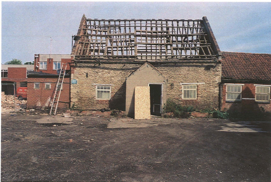
Plate 2 General Site View, showing building with removed roofing, looking north
