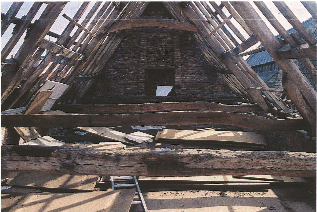
Plate 8 Detail of fireplace, looking east
