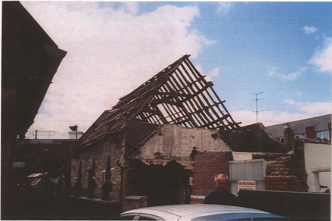
Plate 1 General Site View, showing building with removed roofing, looking northwest
