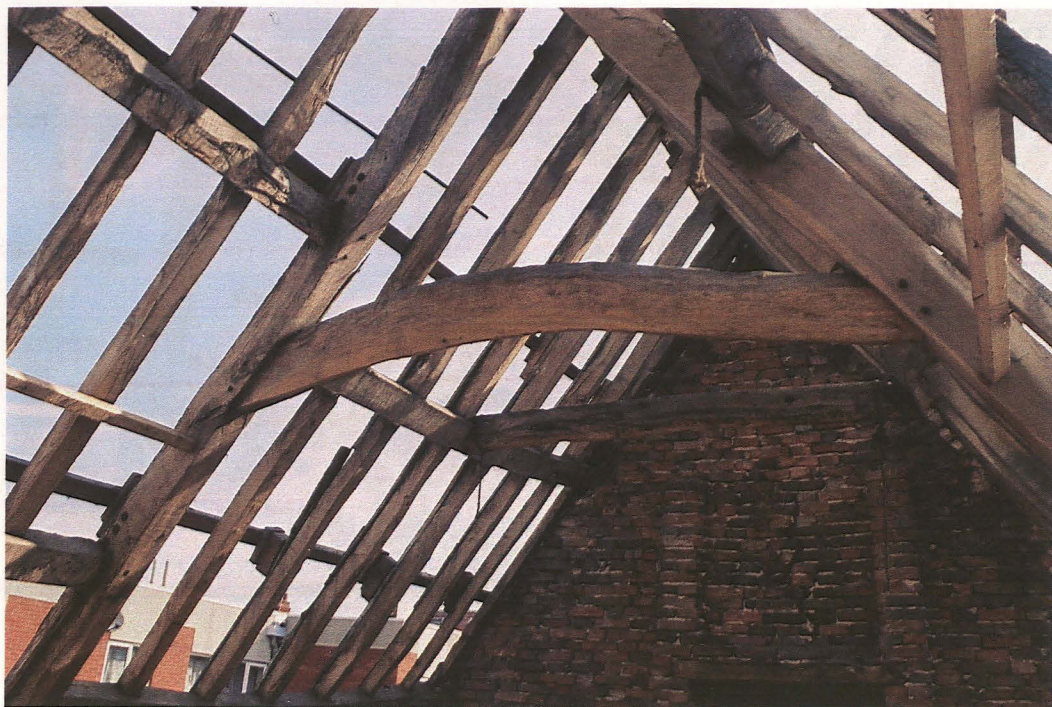
Plate 5 Detailed view of pegging of roof timbers, looking northeast
