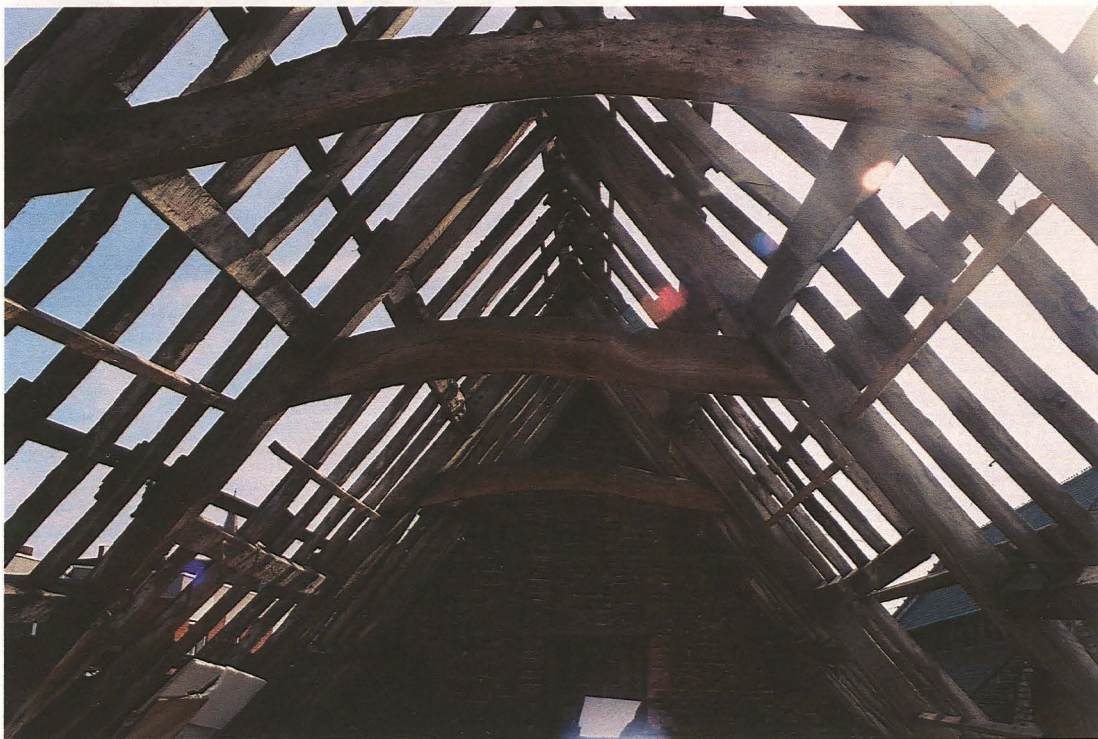
Plate 4 Detailed view of roof trusses, looking east
