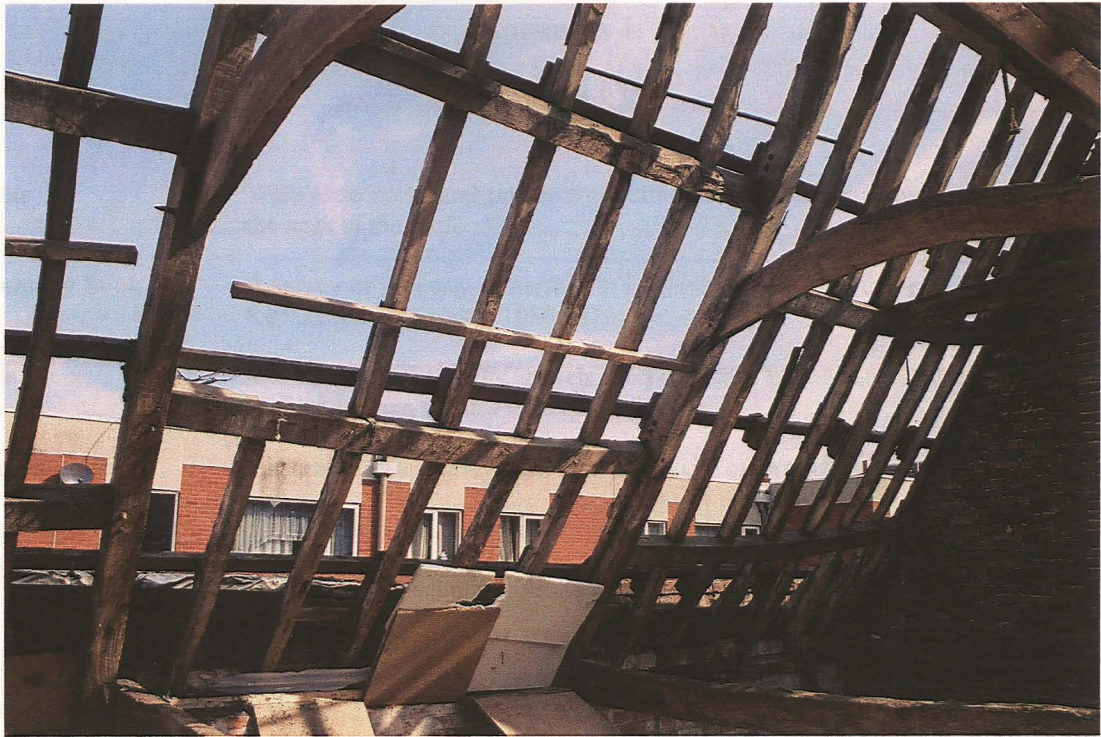
Plate 7 Detail in variations in roof timbering indicating possible former location of dormer window, looking northeast
