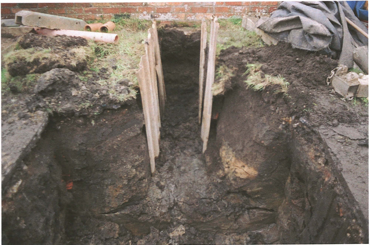
PI. 20 Excavations for linkage and manhole F3 off Dukes Head Lane
