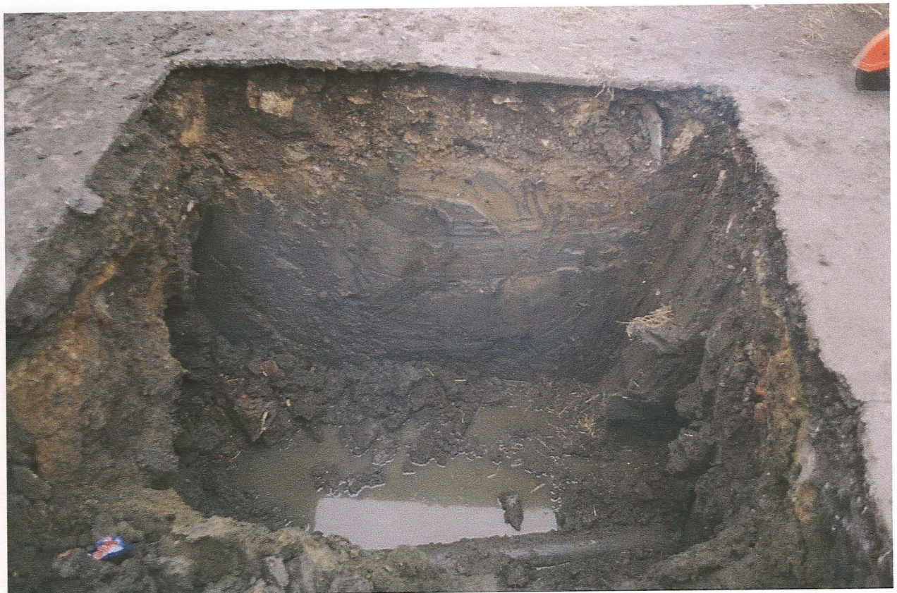
Pl. 7 Excavations for manhole B2 on Church Lane
