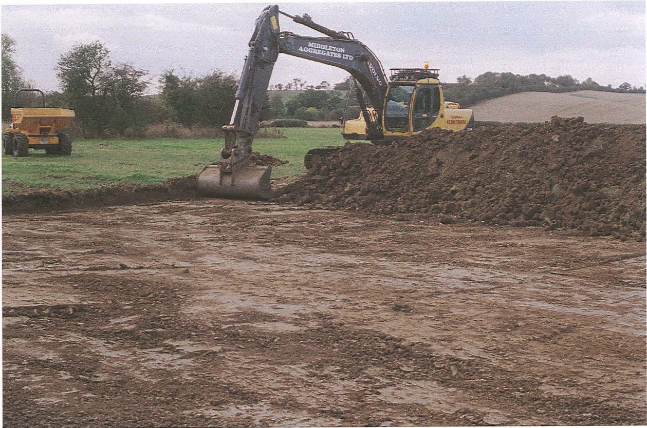
PI.3 Looking north across area being stripped for developers compound
