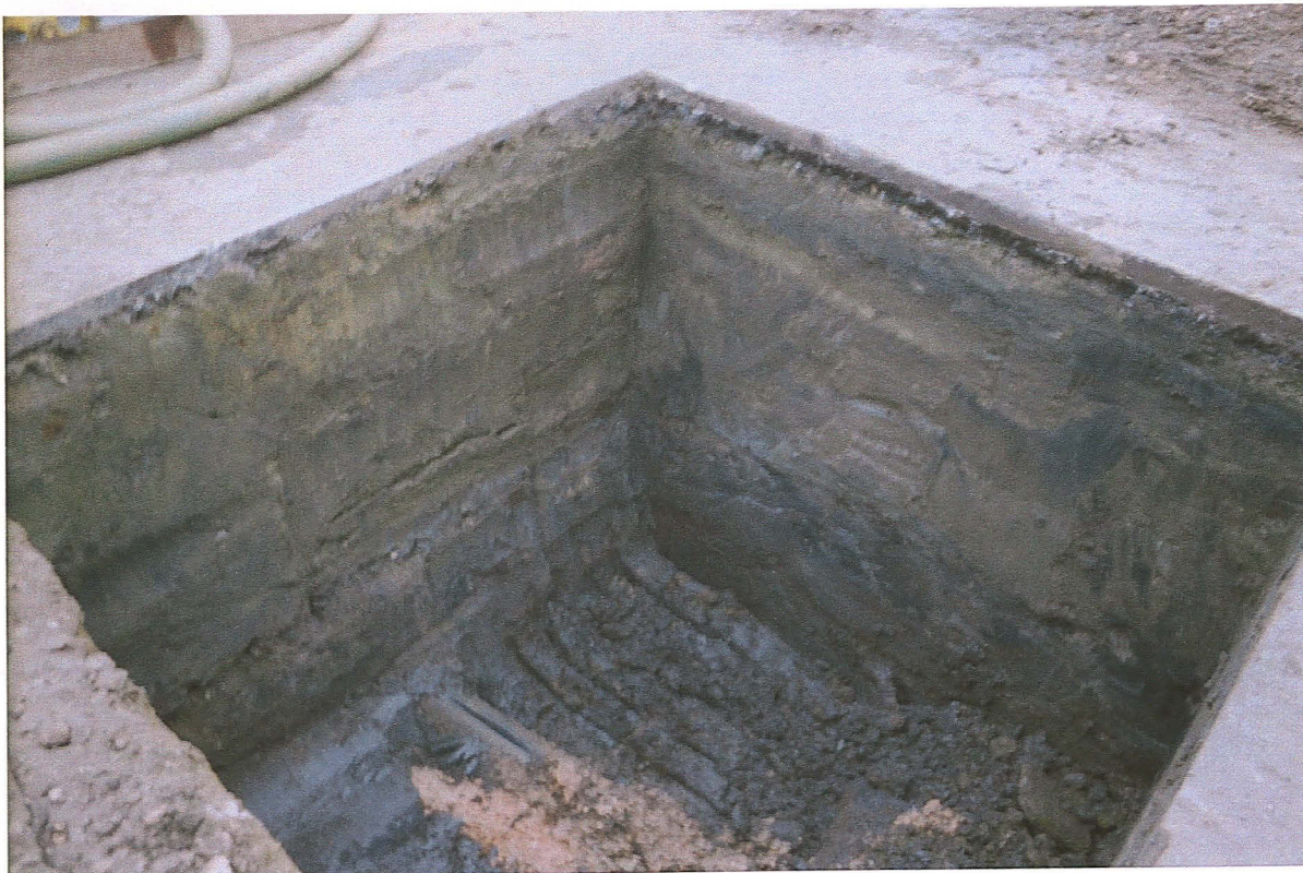
Pl. 16 Excavations for Manhole F7 on West Keal Road
