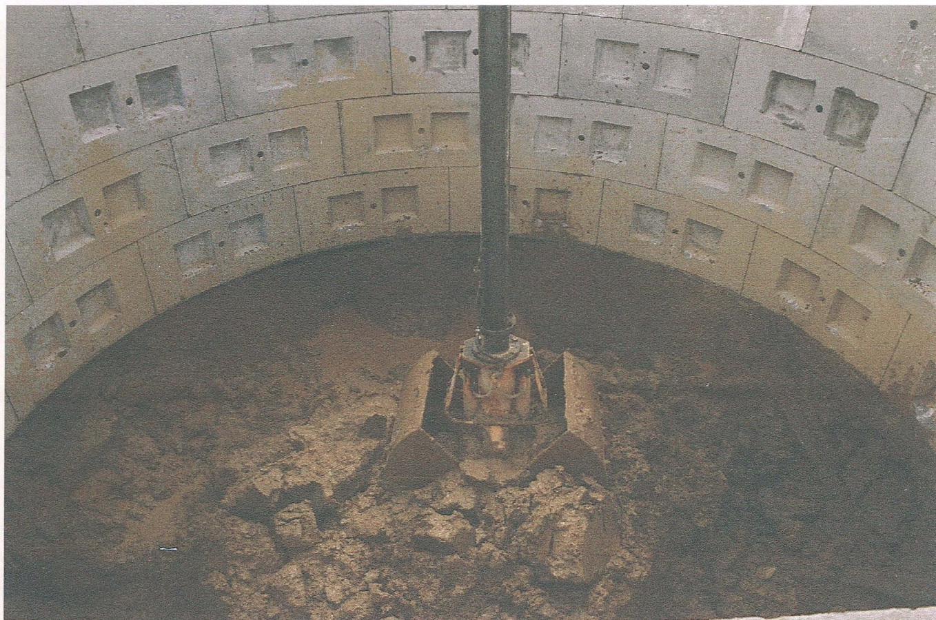
Pl. 3 The grab bucket excavating the chamber for the caisson pumping station
