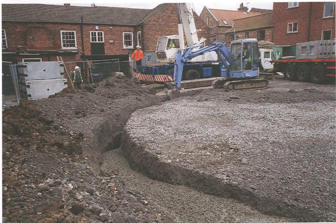
PI.2 Initial trenching prior to the excavation and installation of the caisson pumping station
