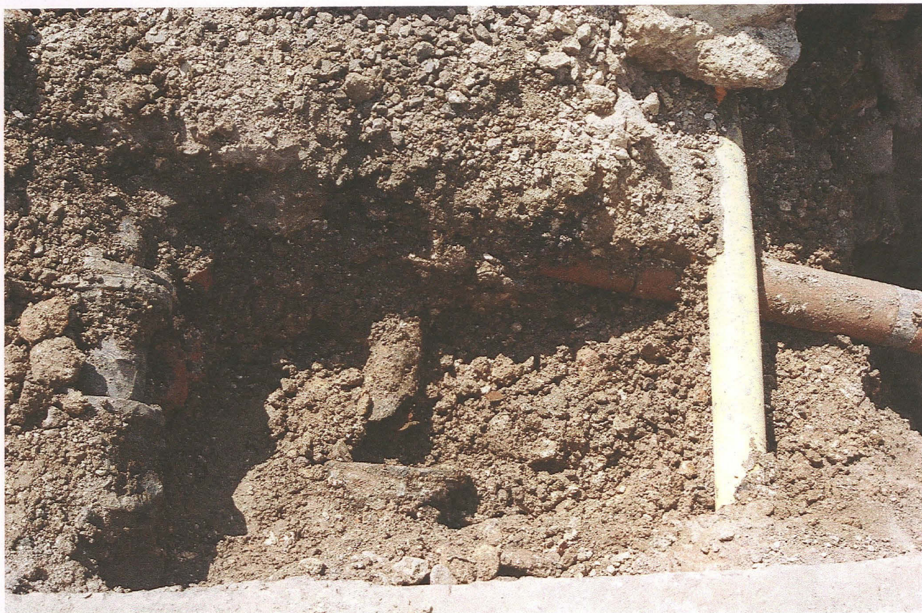
Pl. 13 Looking east at the excavations in Edward Street with five services pipes in a 2.00m wide area
