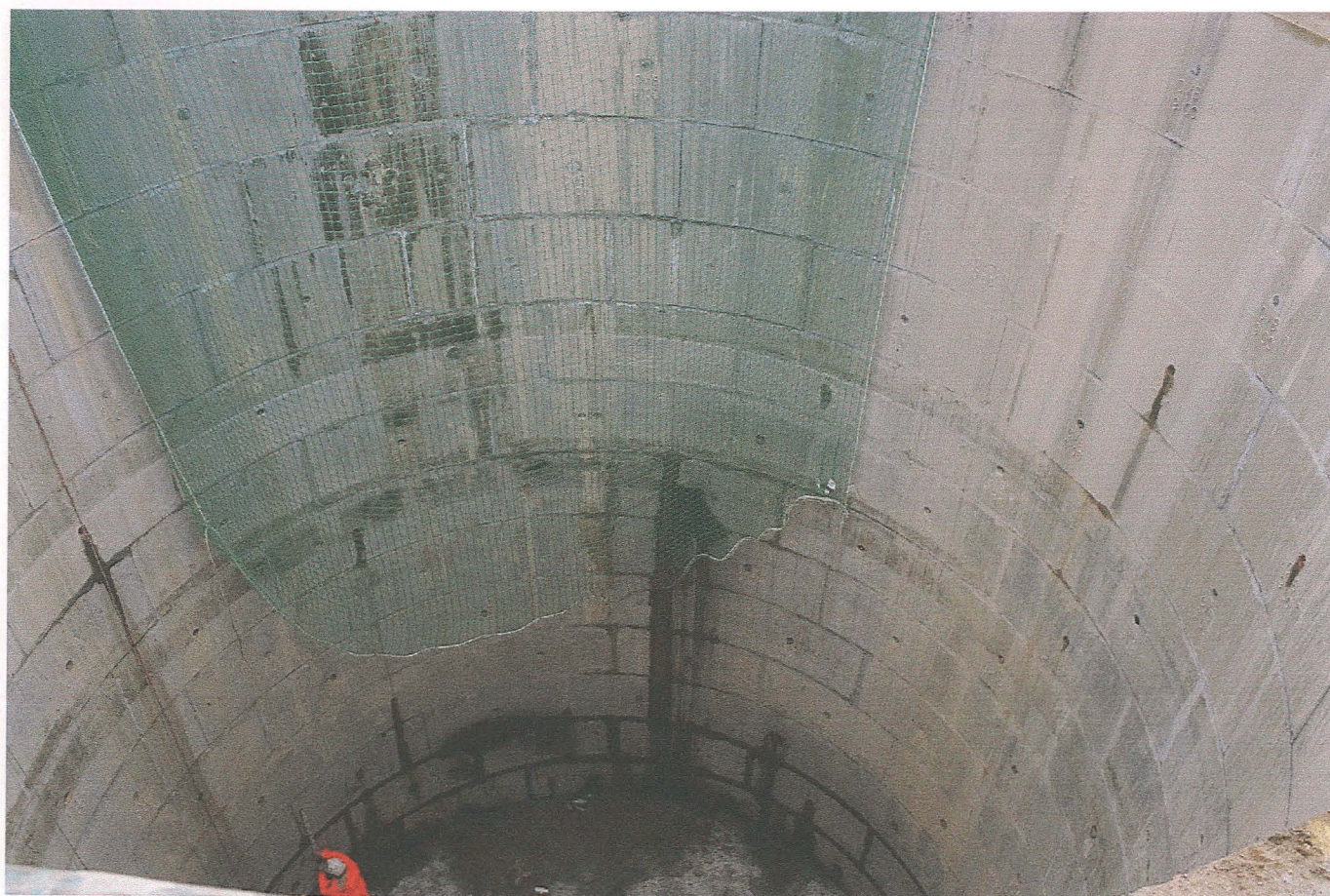
Pl. 4 The completed 14.00m deep pumping station chamber
