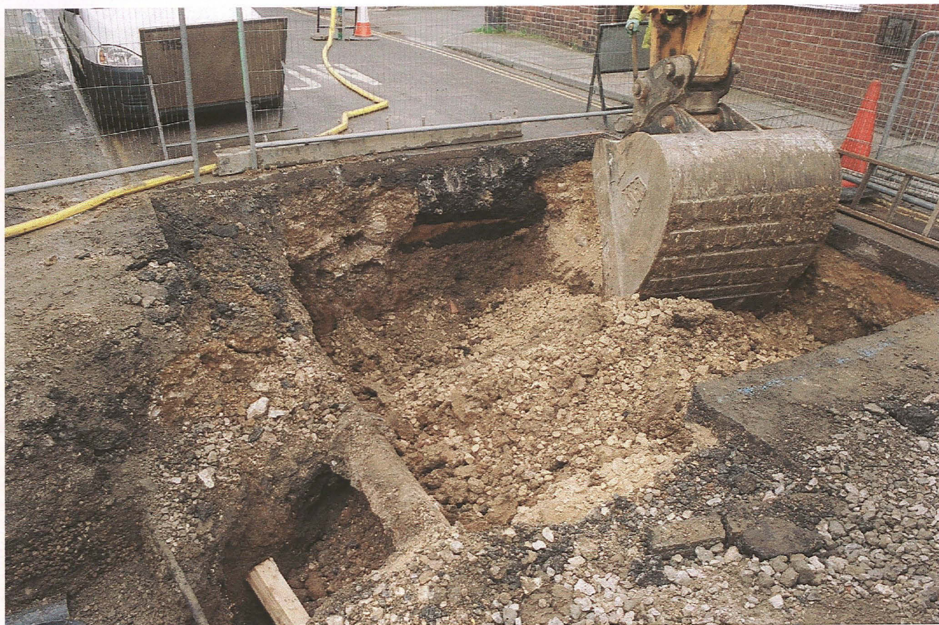
Pl. 7 Services and modern build-up in the excavations for the manhole directly north of the entrance to the Greyhound public house car park
