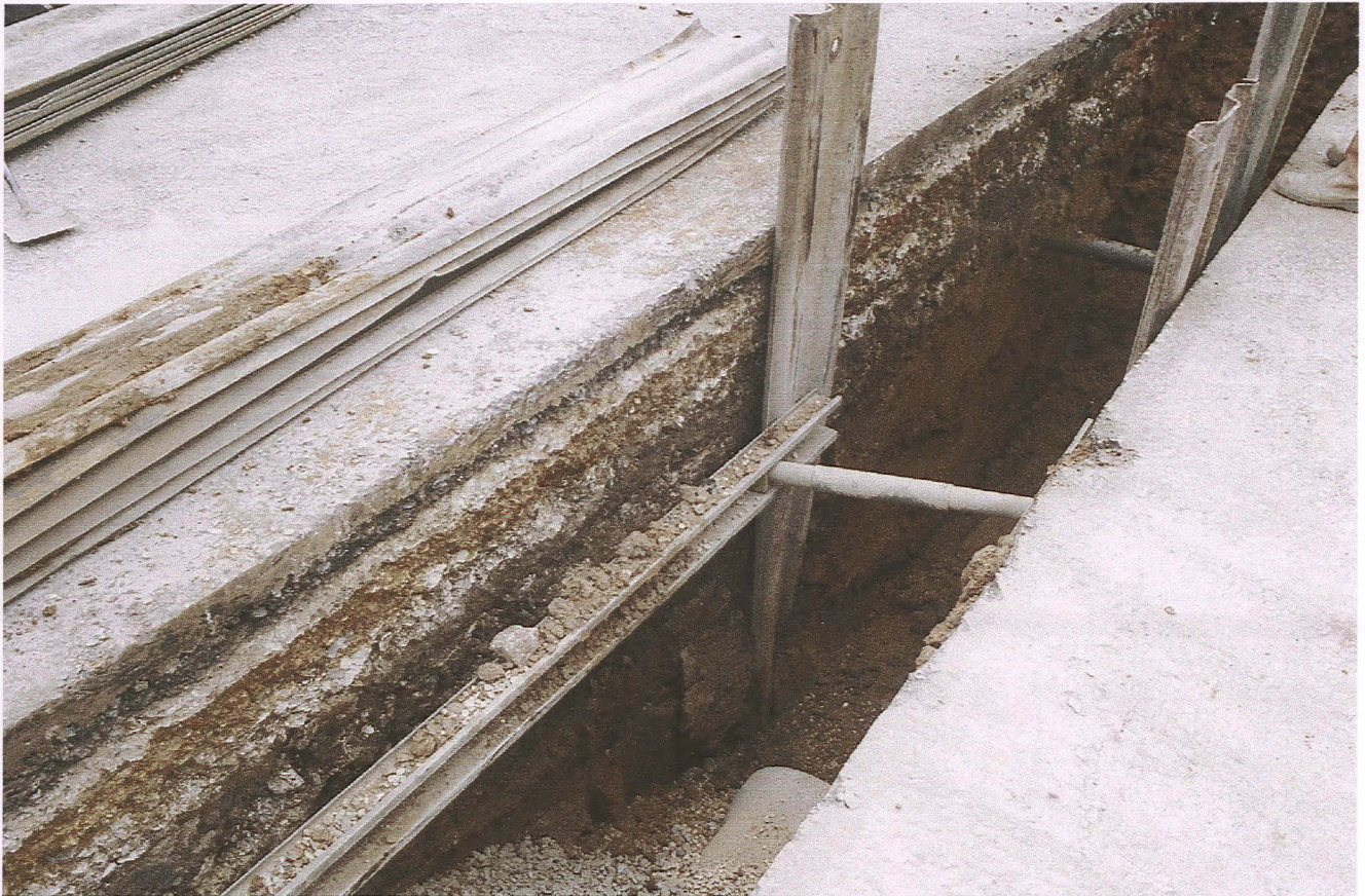
Pl. 15 Modern road build-up and natural clay noted in the excavations along Ugate
