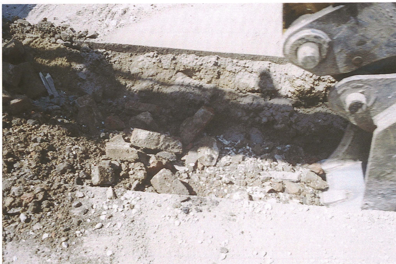
Pl. 12 Rubble and road build-up material noted along Edward Street
