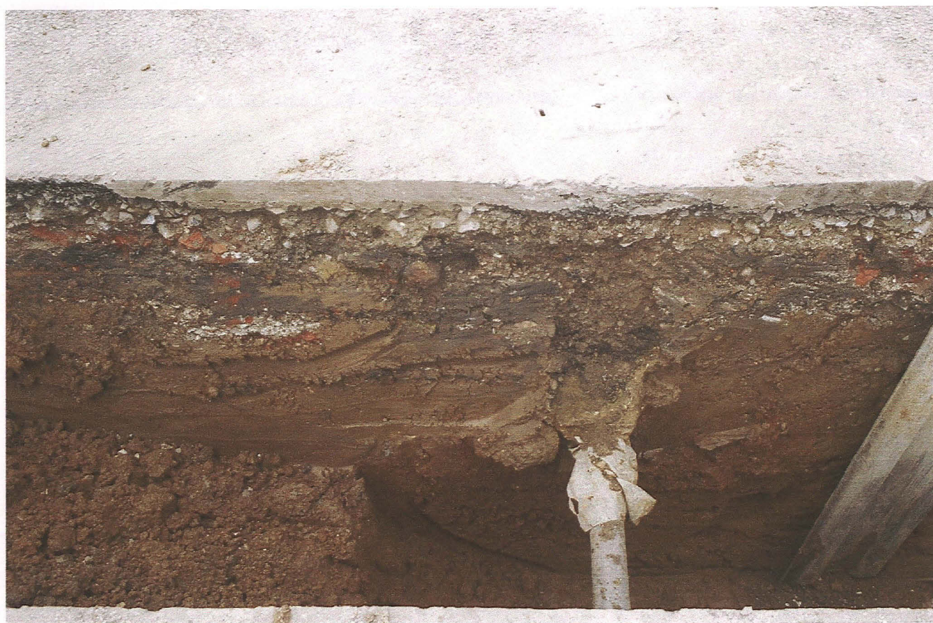
Pl. 10 Services, modern road build-up and undisturbed clay in the excavations along Edward Street
