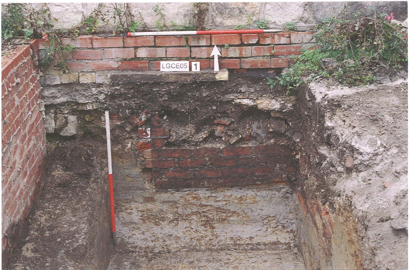
Pl. 4 The northern face of Trench 1 showing modern underpinning. Scales 1.00m
