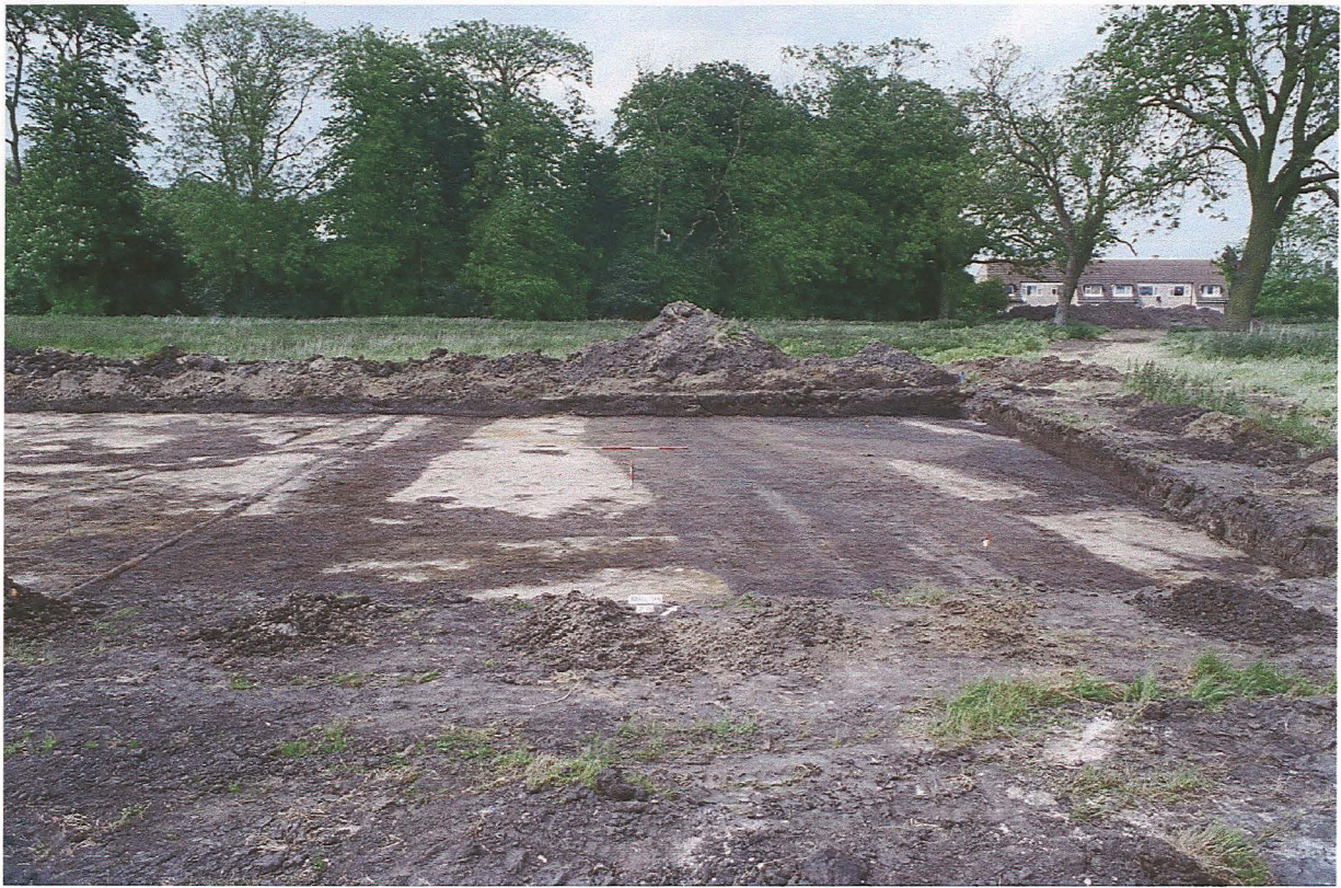
Pl. 5 Area 1b, eastern half, looking north. Scales 2m.
