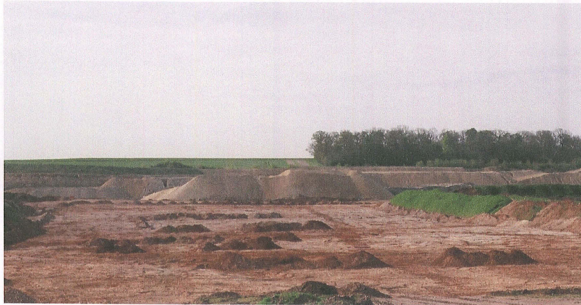
PL. 2 General view of site looking south
